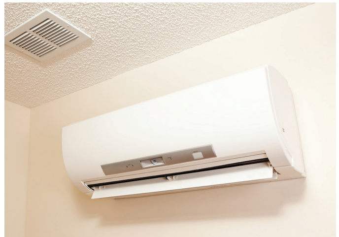
A wall-mount mini-split heating and air conditioning unit.
