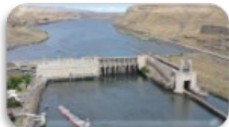
Lower Monumental 6 Units 930 MW*
