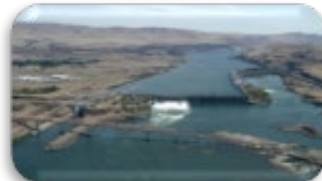
The Dalles 22 Units 2,080 MW*
