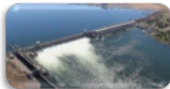
McNary 14 Units 1,120 MW*
