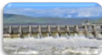
John Day 16 Units 2,480 MW*
