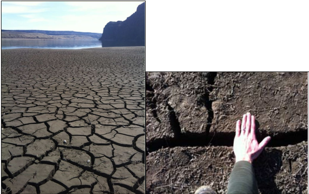
7019 7020 Figure 3-228. Polygonal Crack Formation, Wanapum Drawdown, 2014 7021 Source: DeLeon (2014)
