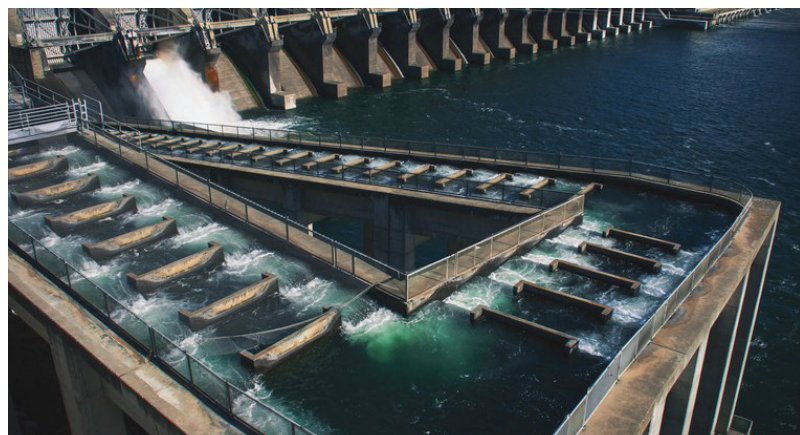
The fish ladder at John Day Lock and Dam that allows adult fish to migrate upstream of the dam.
