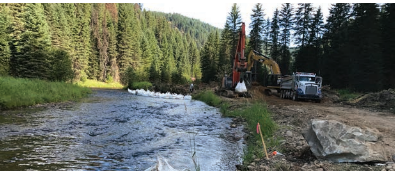
For almost 100 years, the Crooked River in north central Idaho’s Nez Perce-Clearwater National Forest was trapped in a tangle of turns caused by dredge mining in the river and its floodplain. This tributary habitat restoration project removed mine tailings which blocked the stream for decades, and restored the natural floodplain and river flows.
