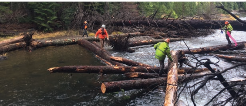
Yakima County, Washington. Adding wood structures reduces stream velocity and pushes water into streamside floodplains and wetlands, many of which have been disconnected for decades as a result of past forest practices.
