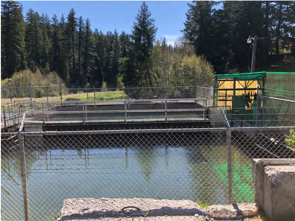
Photo 18. Looking southeast across the hatchery pond.
