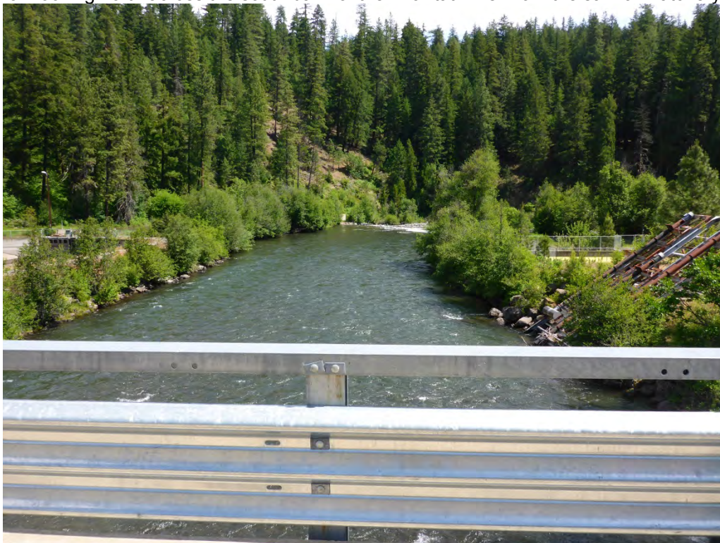
Photo 6. Looking northeast at downstream section of Klickitat River from bridge.
