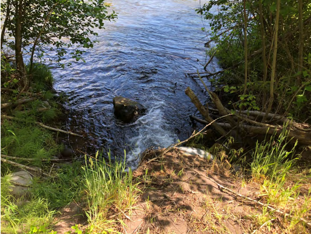
Photo 10. View of culvert where Indian Ford A Spring discharges into the Klickitat River.
