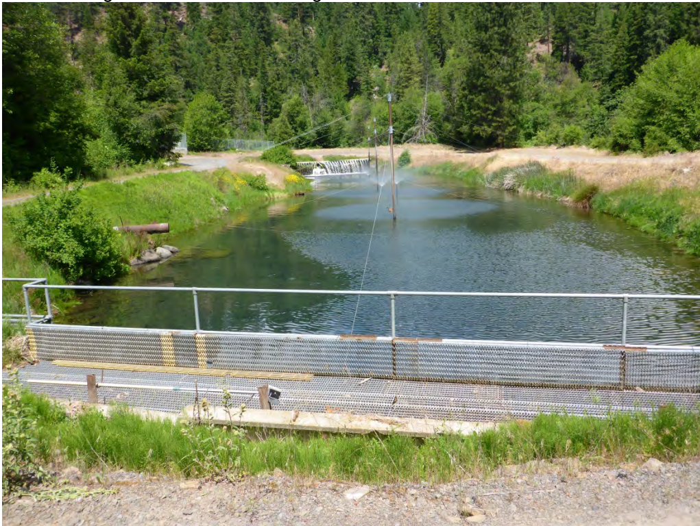
Photo 14. Looking northwest across Rearing Pond 24.
