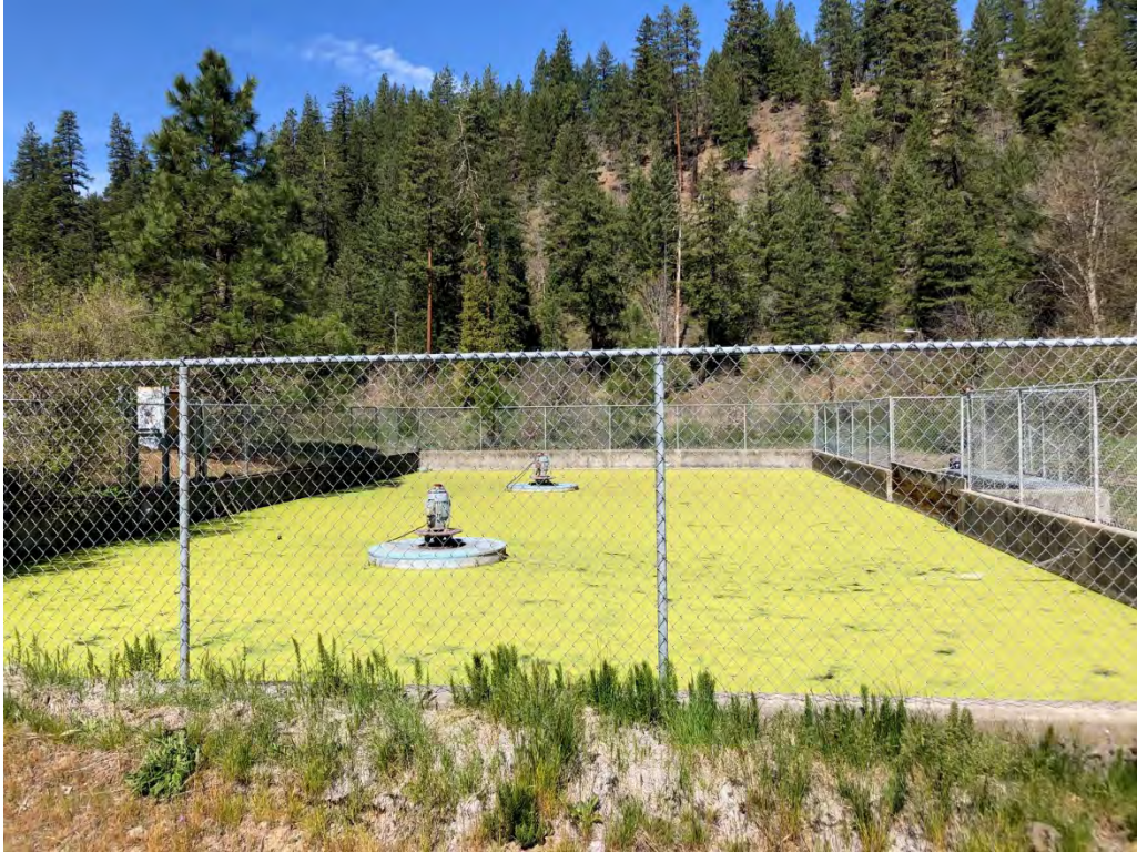
Photo 19. Looking northwest across the pollution abatement pond.
