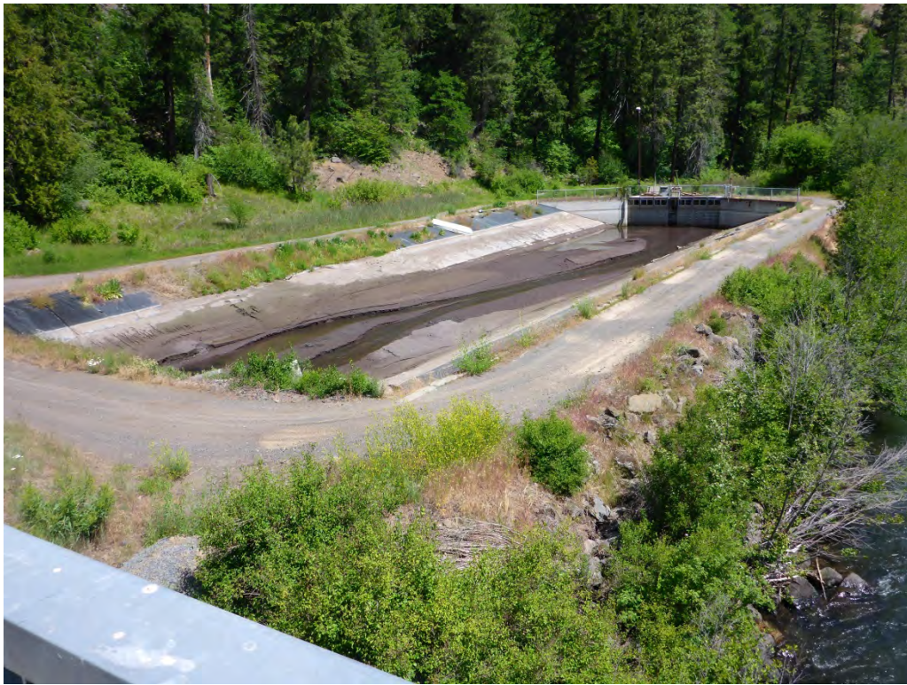
Photo 15. Looking northeast across Pond 25 from bridge.
