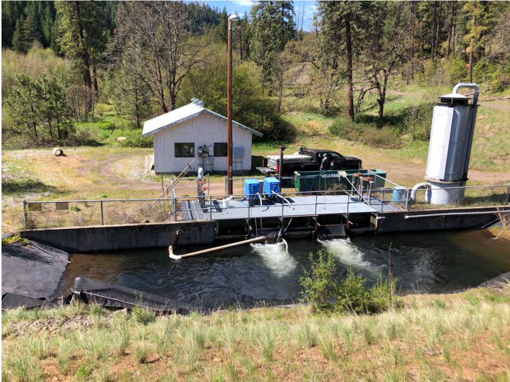
Photo 20. Looking southwest across adult holding pond.
