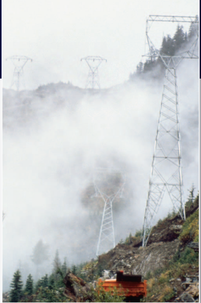
A fire burning under a power line can create a dangerous situation. Stay away from lines if a fire is nearby.
