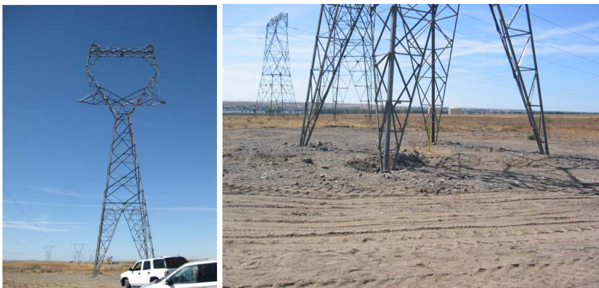
Typical Single-Circuit 500-kV Tower After Construction
