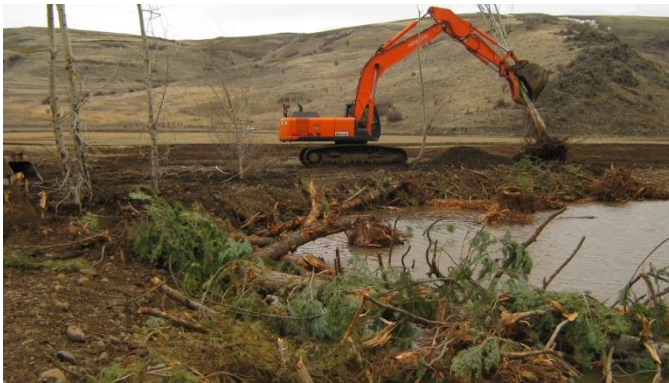
Figure 3 – 300 series Track-mounted excavator
