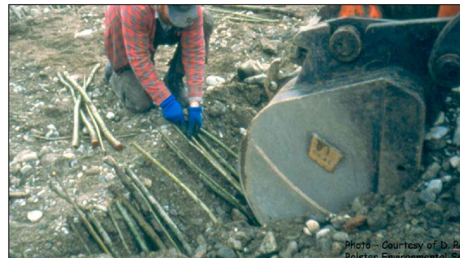
Willow Trench Construction Photo - Courtesy of D. Rolfe, Rolfe Environmental Services
