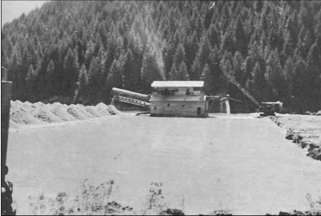
Figure 3-36. Mount Vernon dredge in Crooked River. Dredge processing low-grade placer gravels on Crooked River, about 1938 (Elsensohn 1971:48-7).
