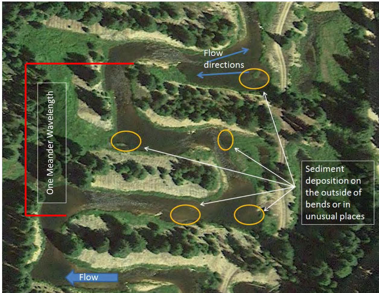
Figure 3-2. Google Earth image of a section of Reach 3 in the tortuous Meanders. Flow eddies at nearly every 90-degree corner. Fish densities, as observed during snorkeling, were very low in this reach. Also, note low potential for woody (evergreen) species interaction with the stream and lack of instream woody debris. Finally, from this picture (July 2012), note minimal shade occurring in and potential to occur on the stream.
