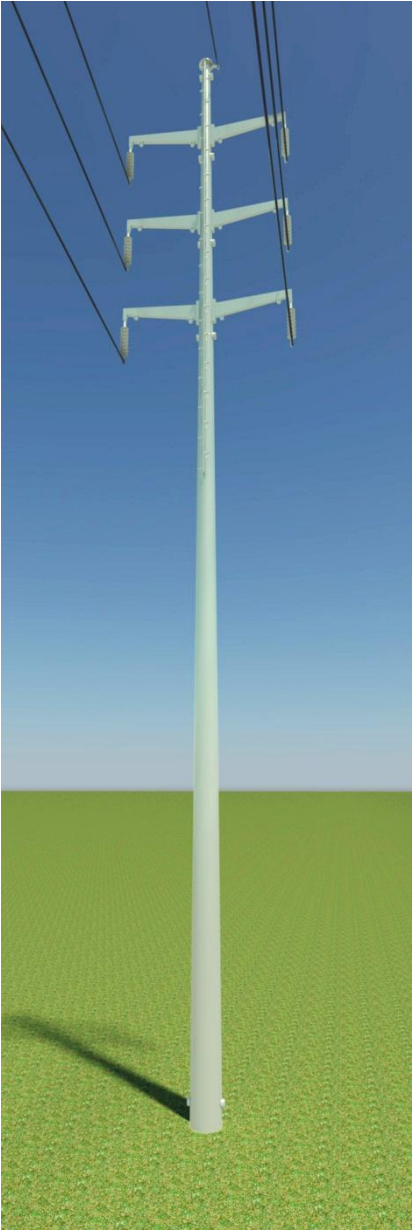
Figure B-3. 3-D model of steel double circuit monopole structures used for photographic simulations
