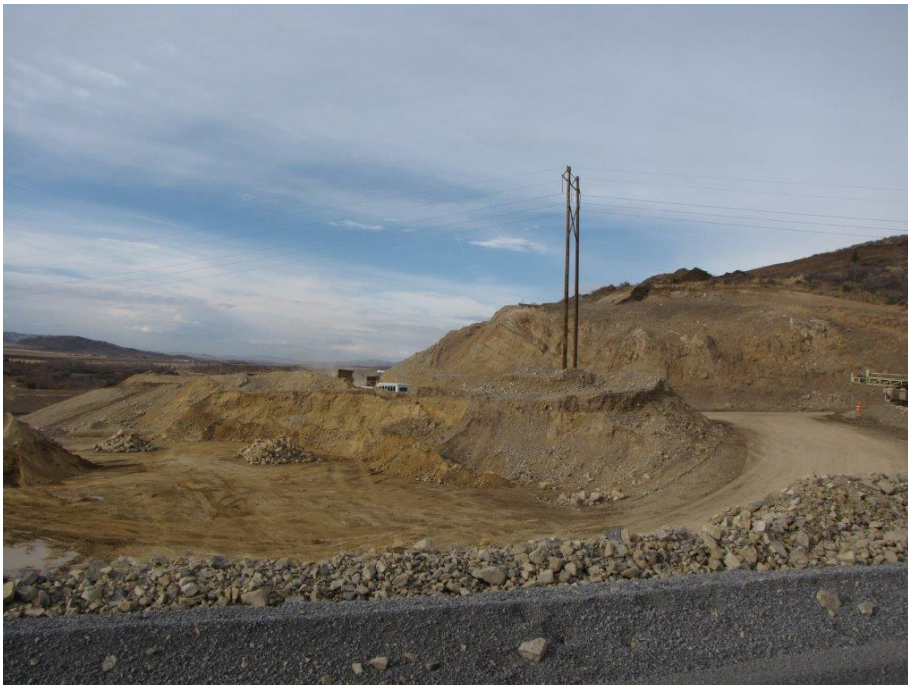
Photo 1. Rocky Mountain Power 138-kV structure within the Blackfoot Bridge Mine area
