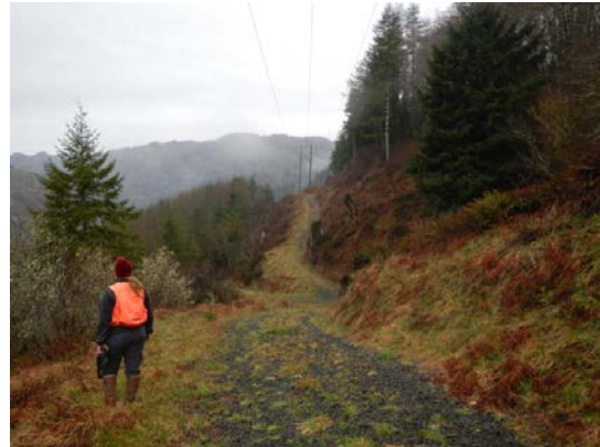
Structure 44/3 (Forest Grove-Tillamook No. 1) in background. Typical access road and disturbed grasses and forbs in the ROW. Adjacent habitats are 40–50 year-old Douglas-fir forest.
