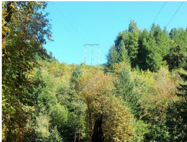
View of transmission line from field at Camp Lane Park
