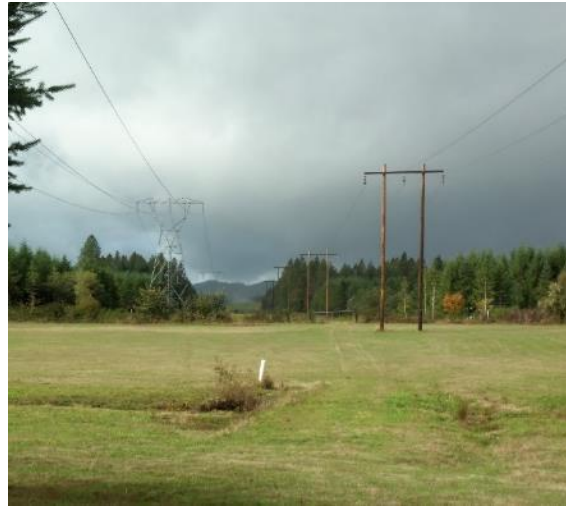
Existing transmission line Line Mile 4—two parallel lines location; BPA's Lane-Wendson No. 2 230-kV lattice-steel tower pictured on left
