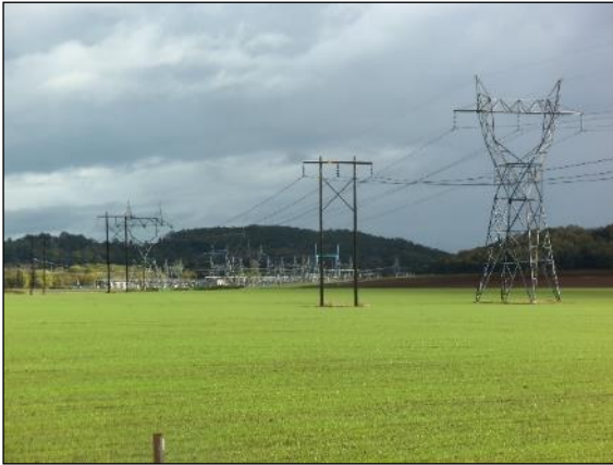
View 1: View from Cantrell Road, looking northeast toward the Lane Substation
