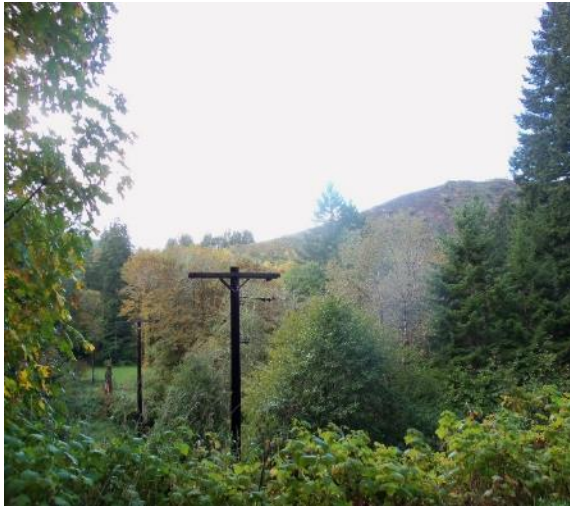
Existing monopole wood structure Line Mile 11—single line location
