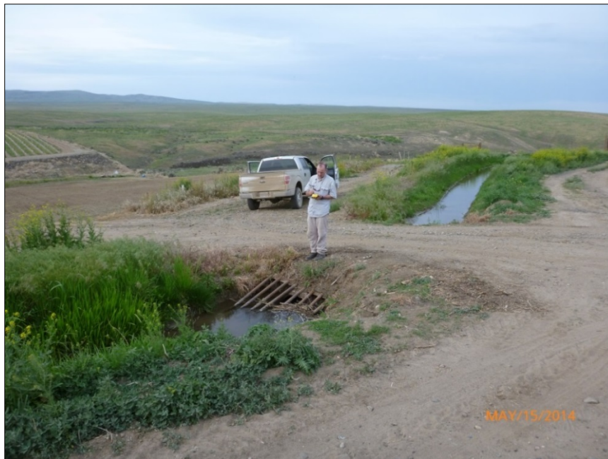
Figure 3.10-5. Photograph shows an existing culvert in an irrigation ditch between Midway-Grandview Structures 23/7 and 24/1 in Line Mile 23 that would not be replaced because existing roads outside the transmission line right-of-way would be used for access . This ditch has been identified as a perennial waterway. (Source: Tetra Tech 2014d)
