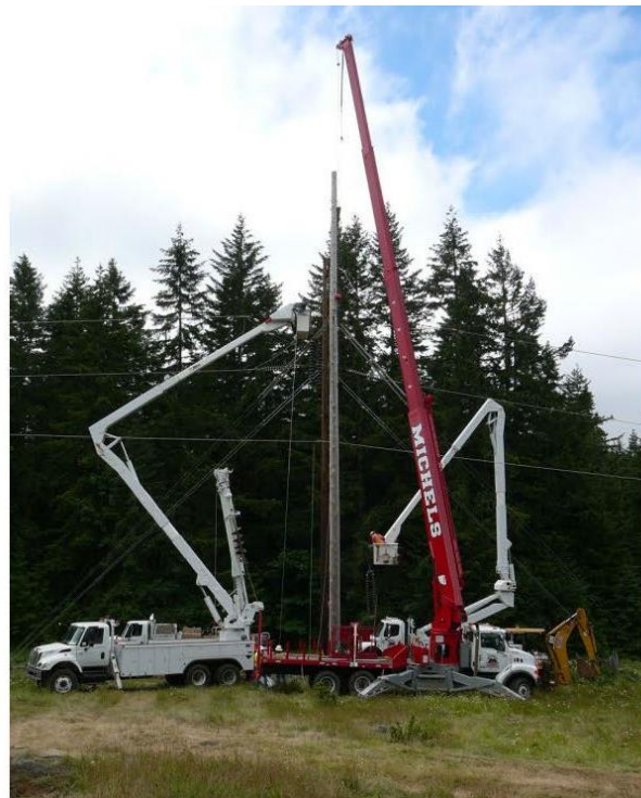
Figure 2-8. Installation of a Wood-Pole Structure
