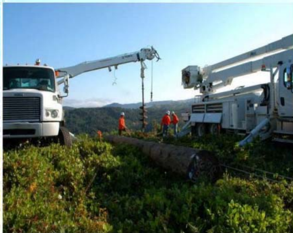
Figure 2-9. Augering a Hole for a Wood-Pole Structure
