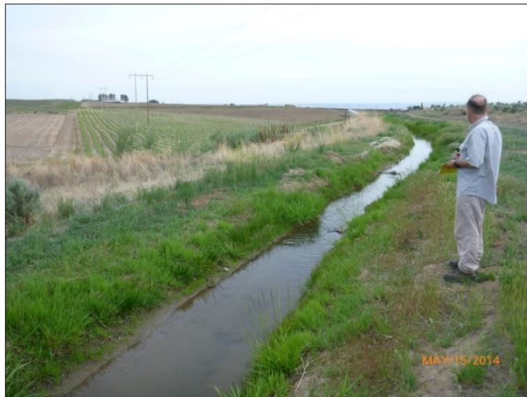
Figure 3.10-3. Photograph shows an irrigation ditch between Midway-Grandview Structures 23/5 and 23/6 in Line Mile 23 where a culvert would not be installed for a new access road crossing because existing roads outside the transmission line right-of-way would be used for access . This ditch has been identified as a perennial waterway. (Source: Tetra Tech 2014d)
