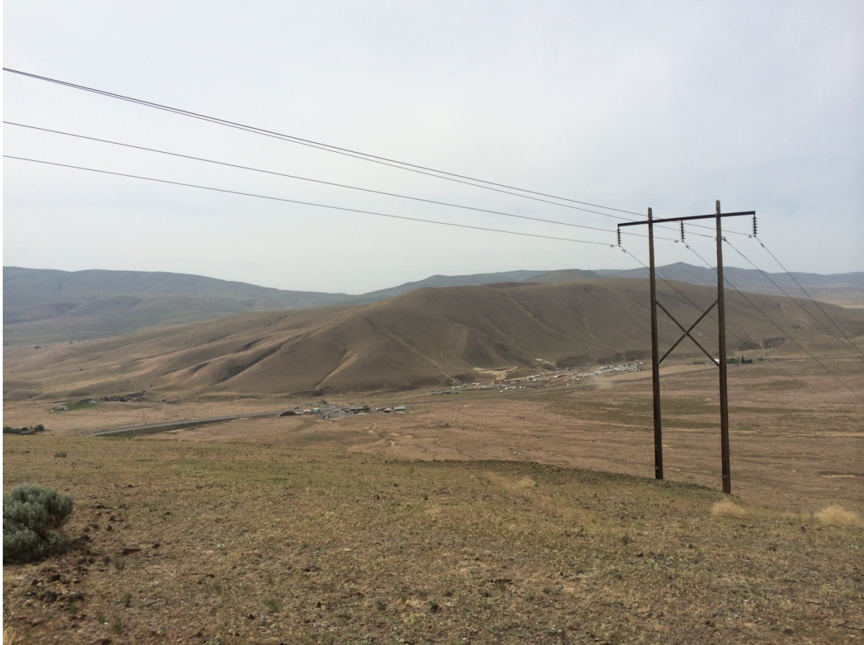
Figure 3.12-1. Photograph of SR 24 from Midway-Moxee Line Mile 8
