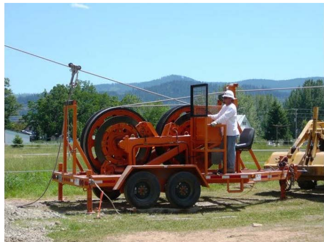
Figure 2-10. Tensioner Pulling Conductor
