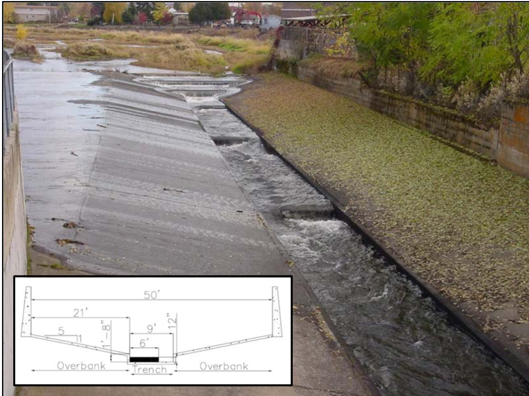
Figure 5. Concrete flume above Roosevelt Street. Insert is example cross section of the concrete flume. (Illustration provided by Tri-State Steelheaders)
