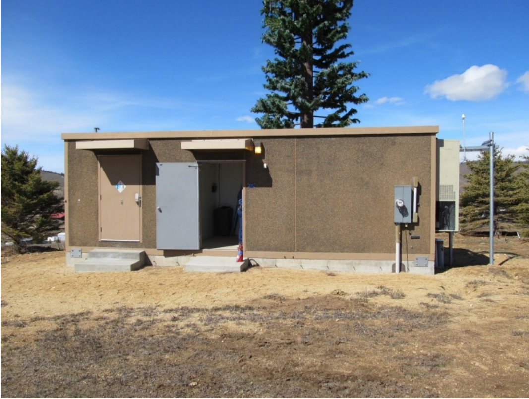
Figure C1-1. Example CTCI Communication Station
