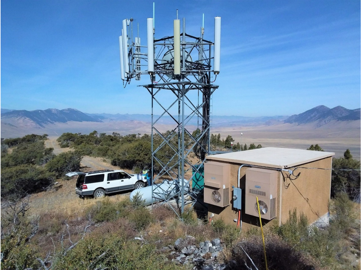
Figure C1-3. Existing Custer Telephone Communication Facility at Willow Creek Summit Looking North
