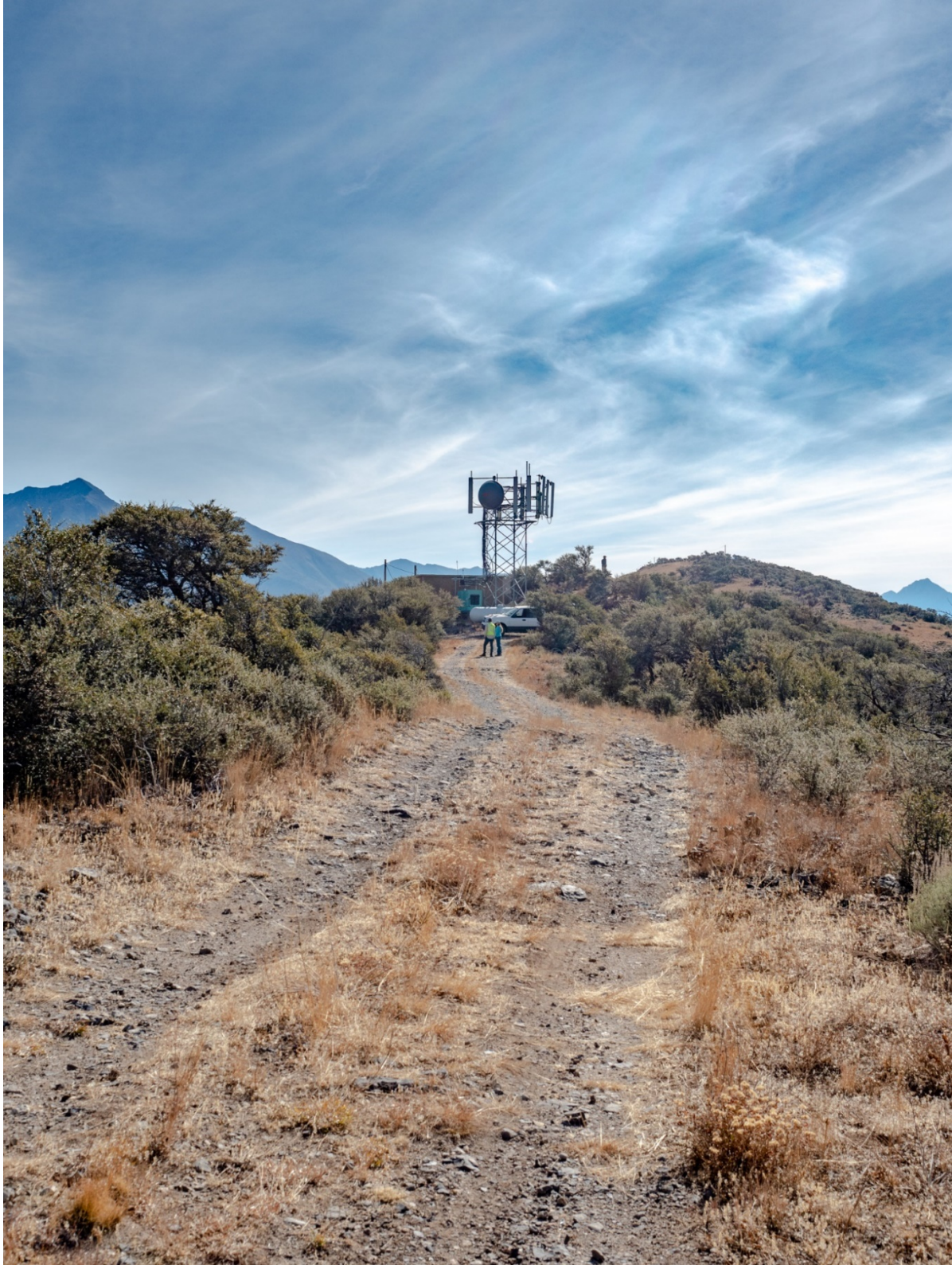
Figure C1-4. Existing Custer Telephone Communication Facility at Willow Creek Summit Looking South
