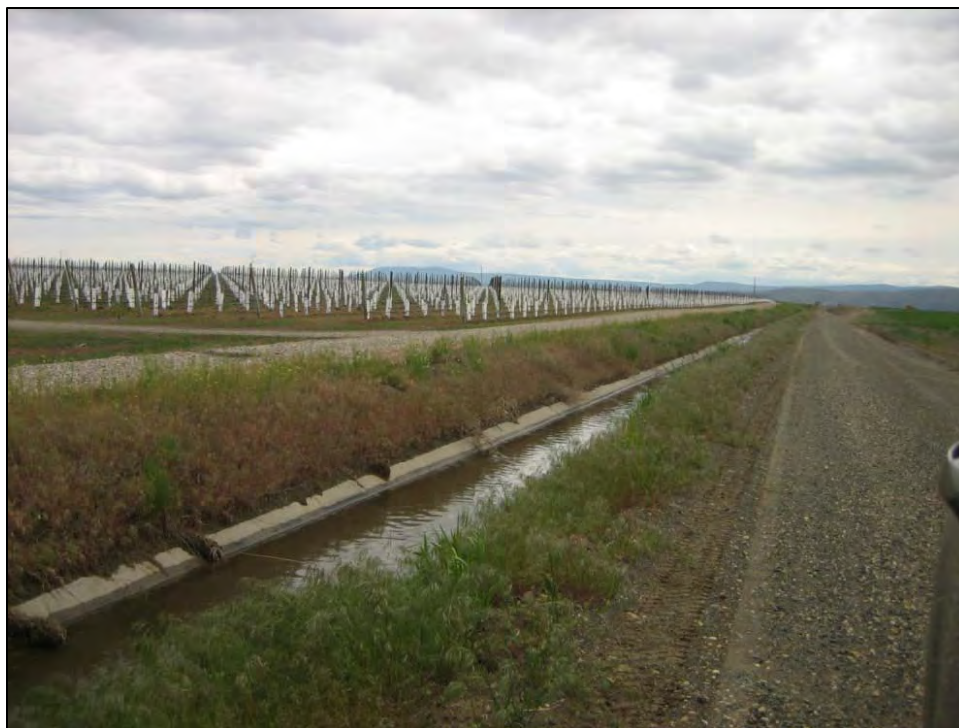
FIGURE 3.4-8 EXISTING IRRIGATION CANAL IN PROJECT AREA
