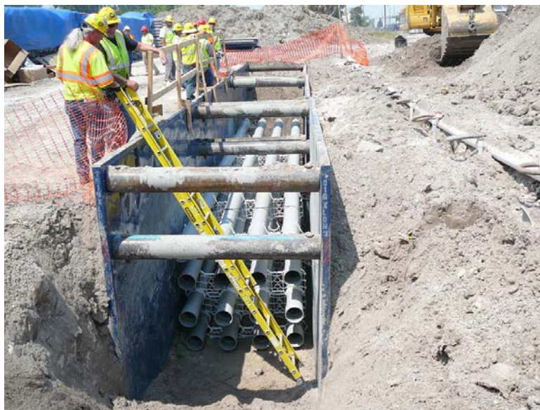
FIGURE 2-9 OPEN CUT TRENCHING (EPRI 2008)
