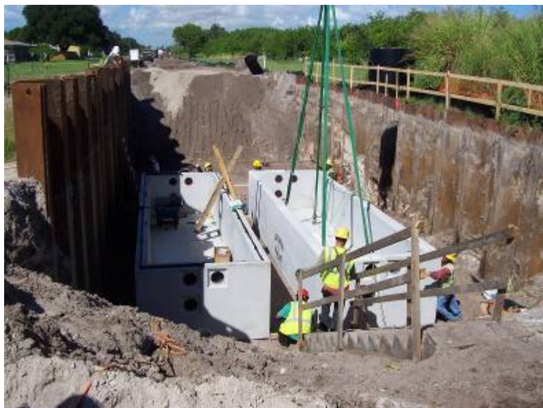
FIGURE 2-11 TYPICAL UNDERGROUND VAULT INSTALLATION (EPRI 2008)
