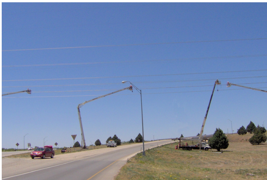
FIGURE 4.7-1 HIGHWAY CONSTRUCTION STRINGING ACTIVITIES
