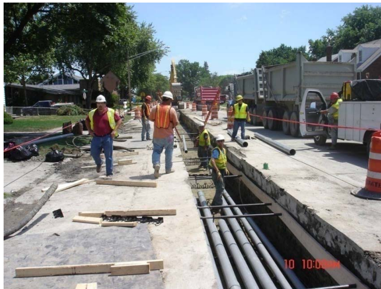
Figure 3-1: Typical Trench Excavation
