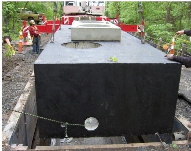
Figure 3-4: Typical Manhole Placement
