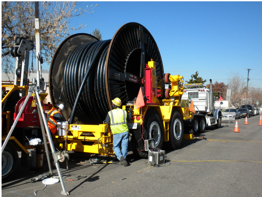
Figure 3-5: Typical Cable Pulling Set up
