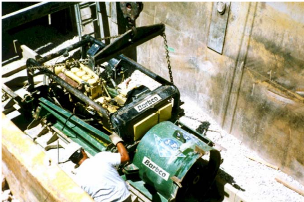
Figure 3-2: Typical Jack and Bore Set-up
