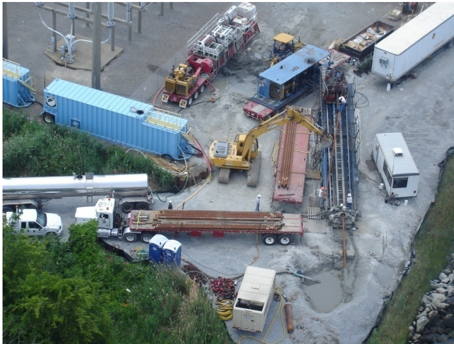
Figure 3-3: Typical HDD Set-up
