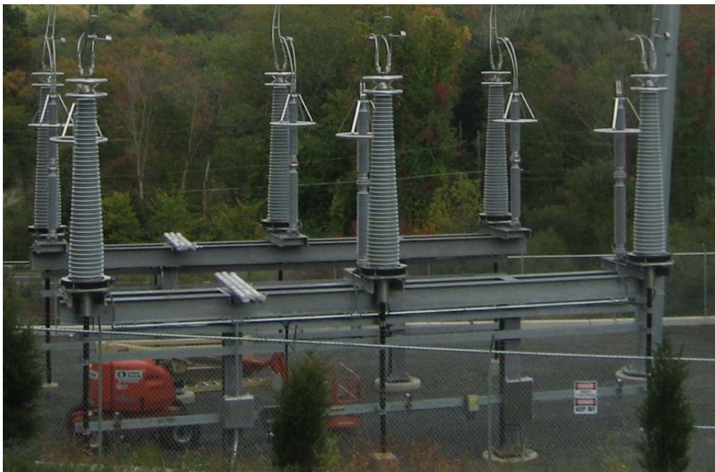
Figure B1-3 Typical 345kV XLPE Termination
