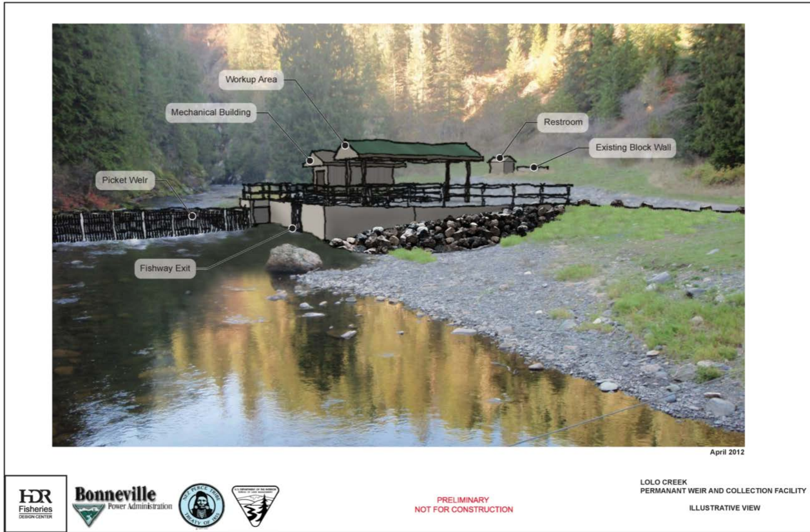
Figure 2-1. Rendering of Permanent Fish Weir with Recreation Elements.
