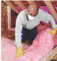
Batt insulation installation
