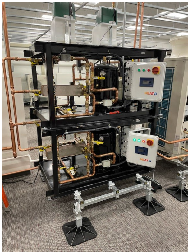
Figure 9. Prototype heat exchanger skids being tested at Mitsubishi Facility.
