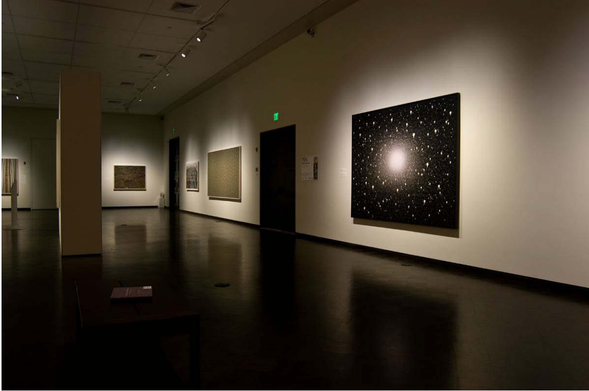
Figure 6. Photo of the gallery with “Running the Numbers” exhibit. All track heads are lamped with Cree “LRP38” lamps (12W LED PAR38, 2700K, 20° beam). (Photo courtesy of JSMA.)
