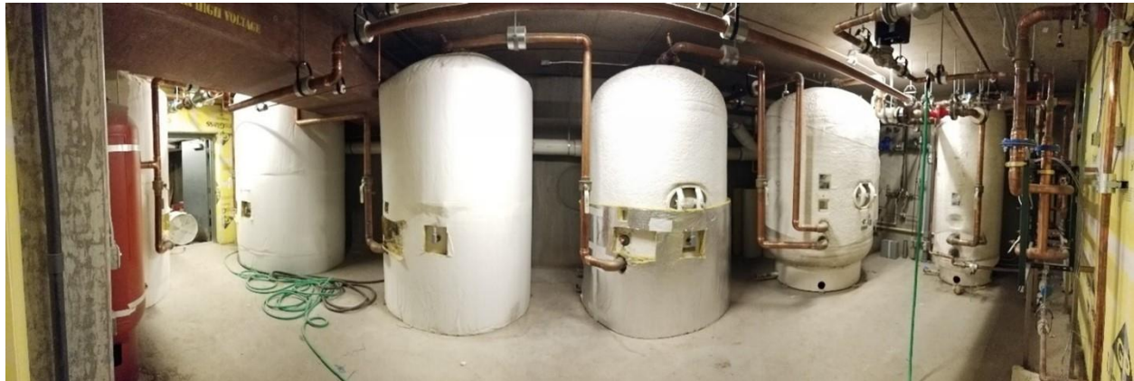
Figure 8. Primary storage tanks during tank and pipe insulation installation
