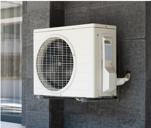
An MSHP side discharge outdoor unit
