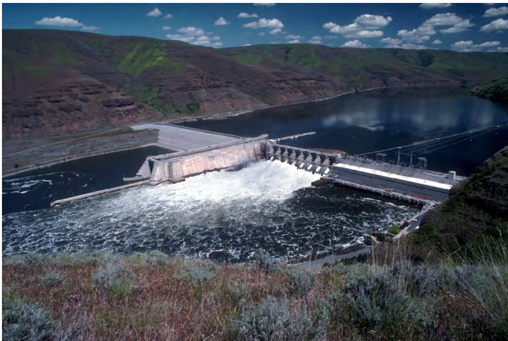
Figure 13. View of Lower Granite Dam.
