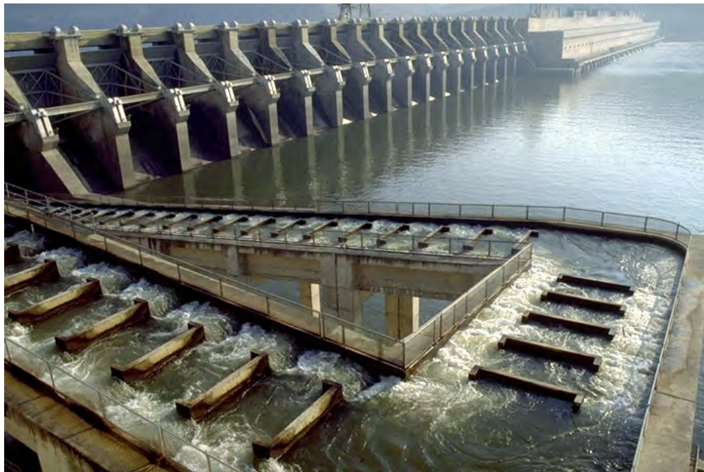
Figure 8. View of John Dan Dam, powerplants, and fish ladder.
