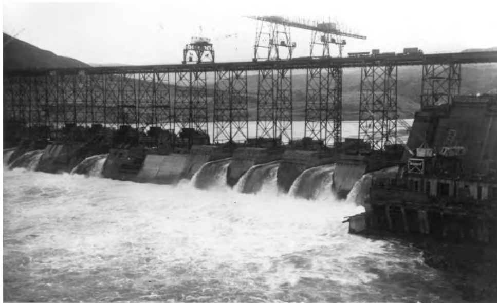
Figure 4. The Grand Coulee Dam, built between 1933 and 1942, is the largest hydroelectric power-producing facility in the United States. The FCRPS Program helps mitigate for the impacts of operating the dam on cultural resources.
