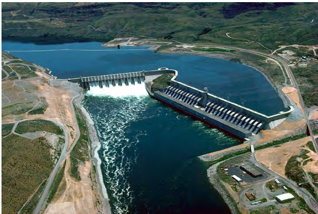
Figure 15. View of Chief Joseph Dam and powerplant.
