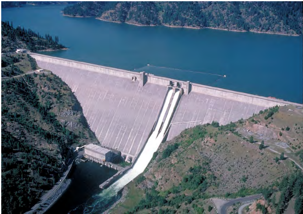
Figure 14. View of Dworshak Dam.
