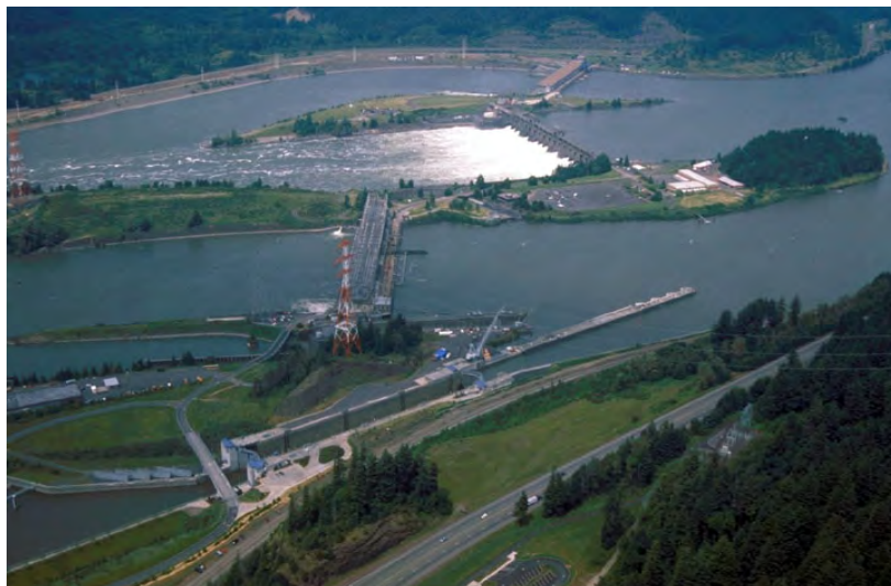
Figure 6. View of Bonneville Dam and powerplant.
