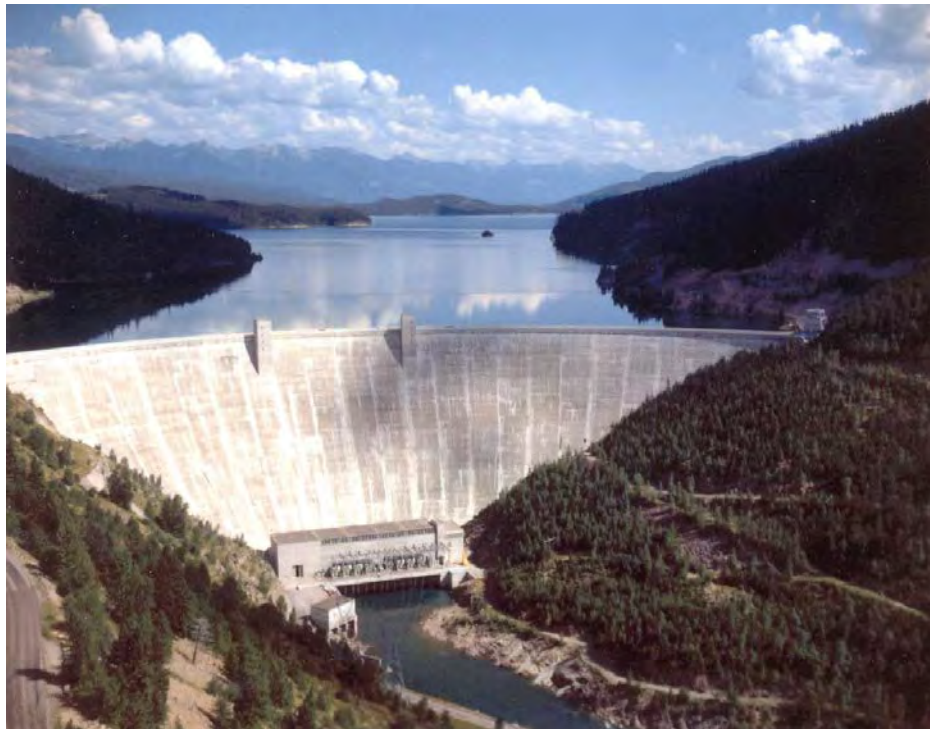
Figure 19. View of Hungry Horse Dam and powerplant looking upstream at Hungry Horse Reservoir.
