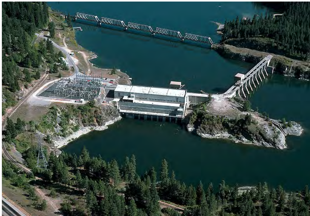
Figure 17. View of Albeni Falls Dam and powerplant.
