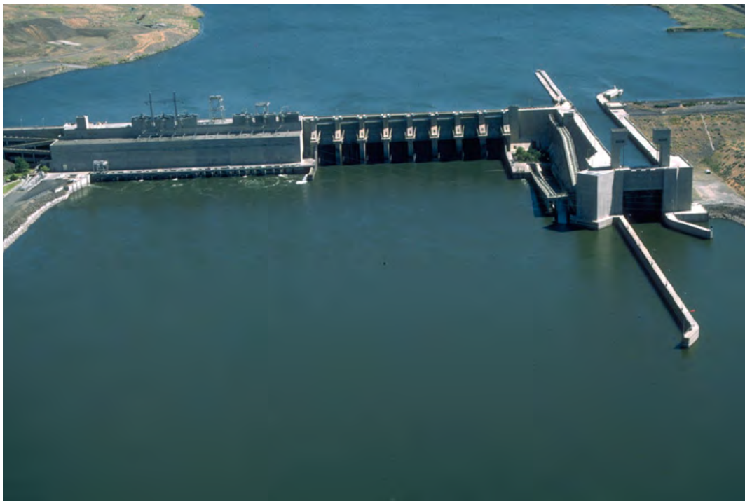
Figure 11. View of Lower Monumental Dam and powerplant.
