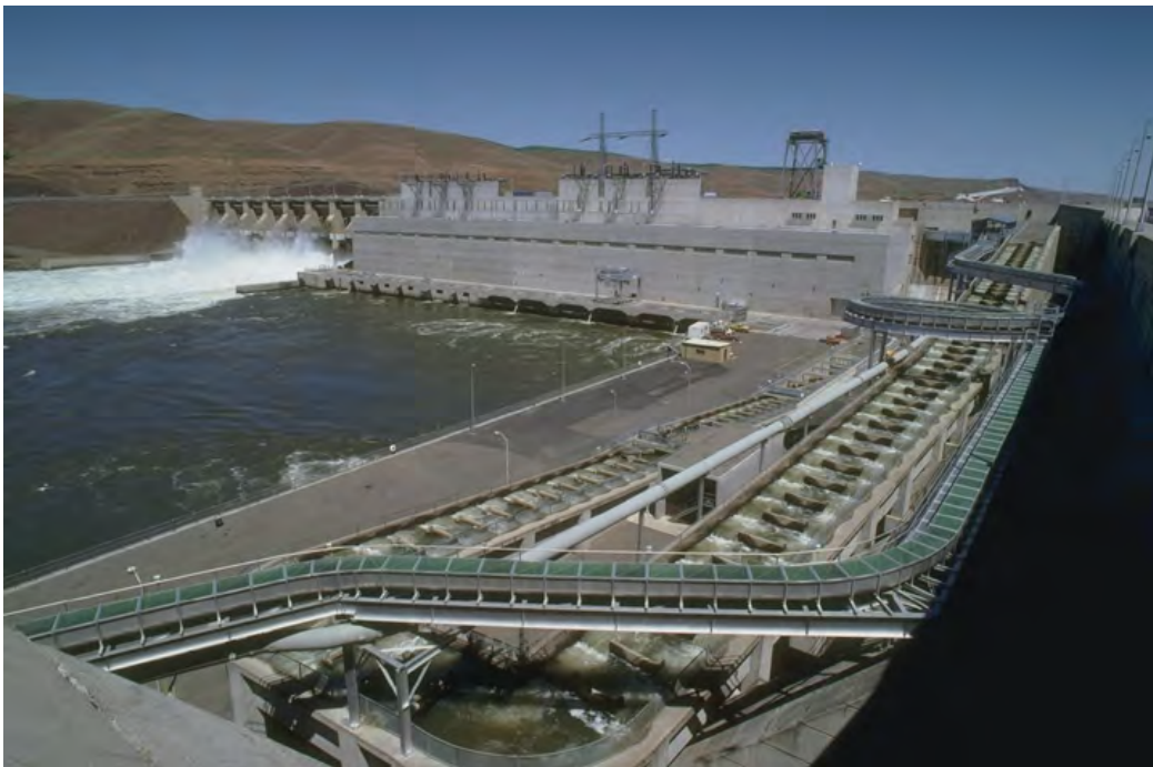
Figure 12. View of Little Goose Dam and powerplant.
