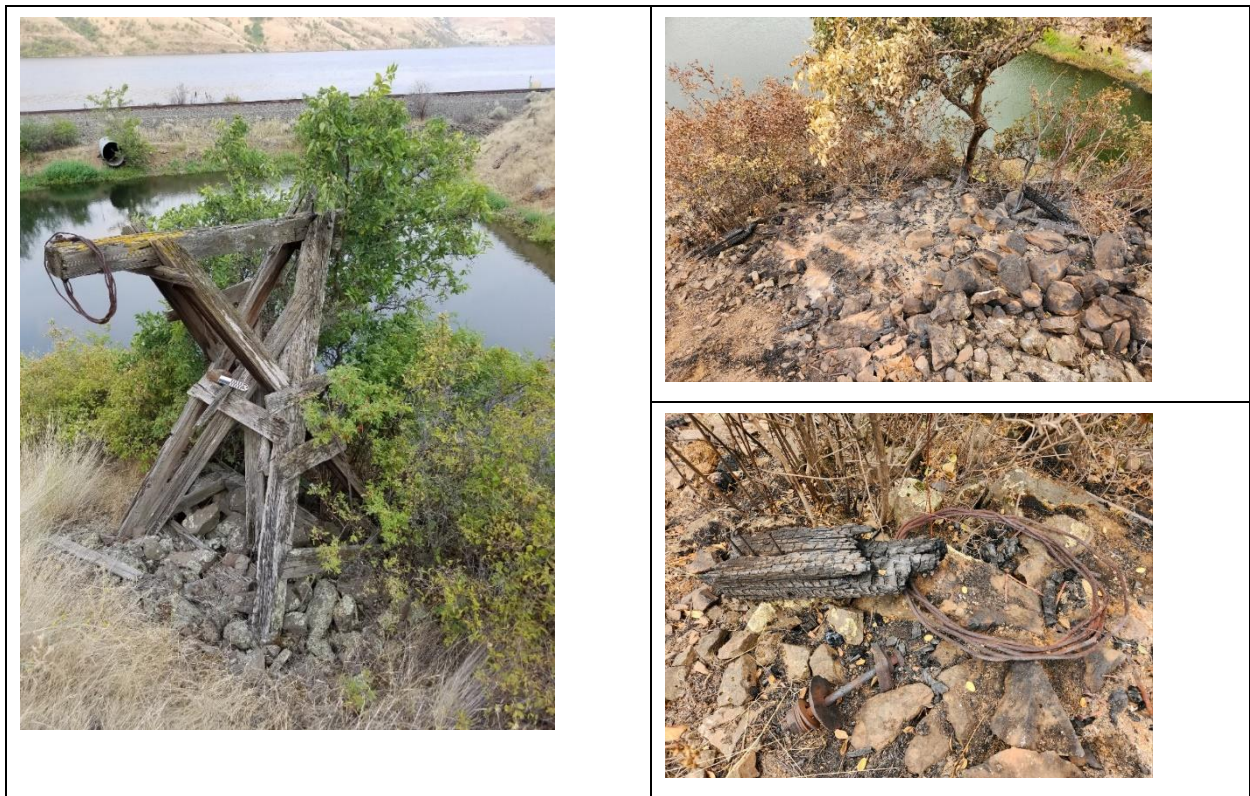
Figure F-6. View of one tower from the NRHP-listed Interior Grain Tramway in July 2018 (left) and August 2023 (right, top and bottom) following the Wawawai Fire.
