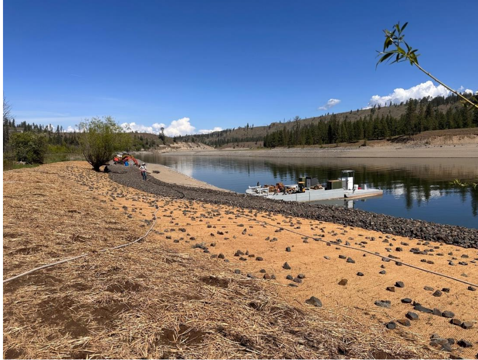
Figure K-6. Concluding phase (Phase III) of the site 45LI377 Stabilization Project, showing the expansive 900-foot-long protection system and barge used to supply materials.
