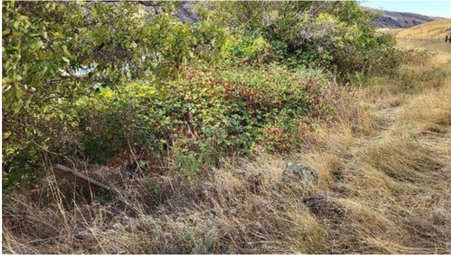
Figure F-5. Site monitoring at 45WT31 by USACE at Little Goose in FY 2023. A sensitive feature at the site is being covered by blackberries, which the PKC Cooperating Group recommended remain in place (even though it is a non-native plant) for erosion control.
