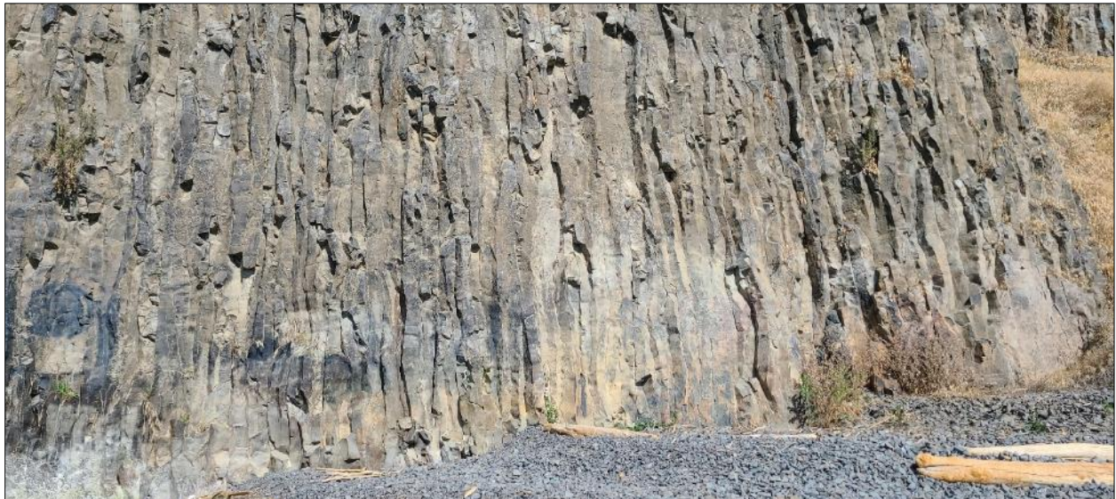
Figure F-2. Overview of site 45BN1753 after graffiti removal (Baird 2023).
