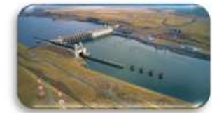
Ice Harbor 6 Units / 695 MW*
