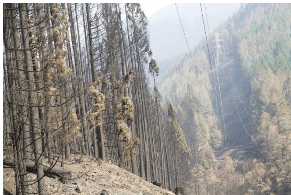
Figure 15 - Looking E showing freezing on N side of ROW
