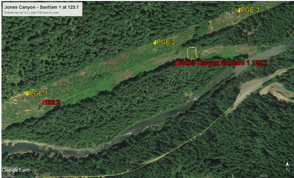
Figure 6 Jones Canyon-Santiam 1 at Structure 123.1 with location of trees shown in yellow, PGE lines to north.
