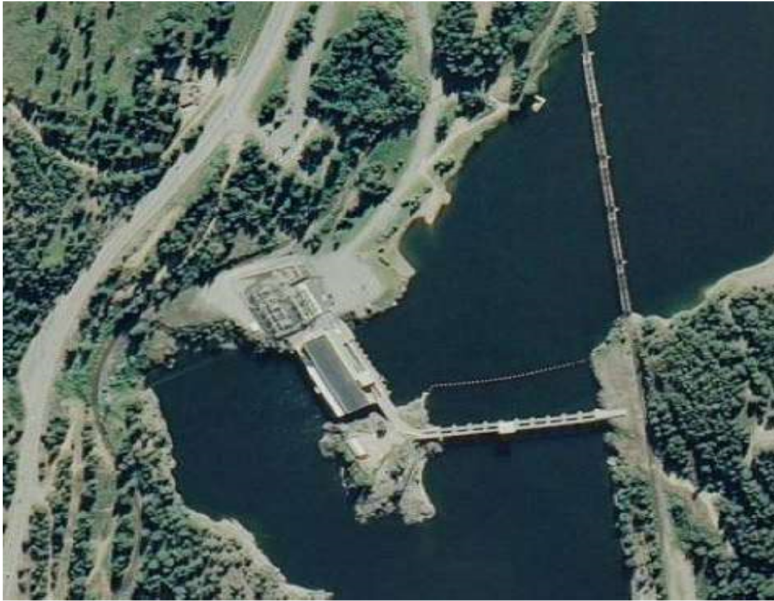
Figure 1-2. Aerial view of Albeni Falls Dam.
