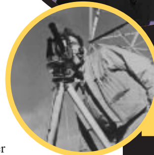
Surveying the first Bonneville-Grand Coulee high-voltage line, 1939.
