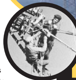
Dead ending the conductor on a river crossing tower for the Bonneville-Vancouver line, 1939.
