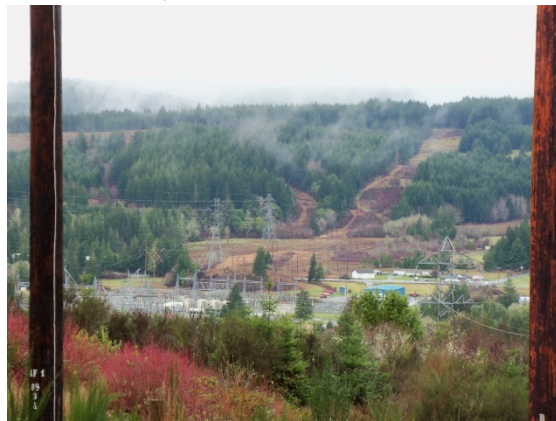
View 6: View of Fairview Substation, looking west from Fairview McKinley Road.
