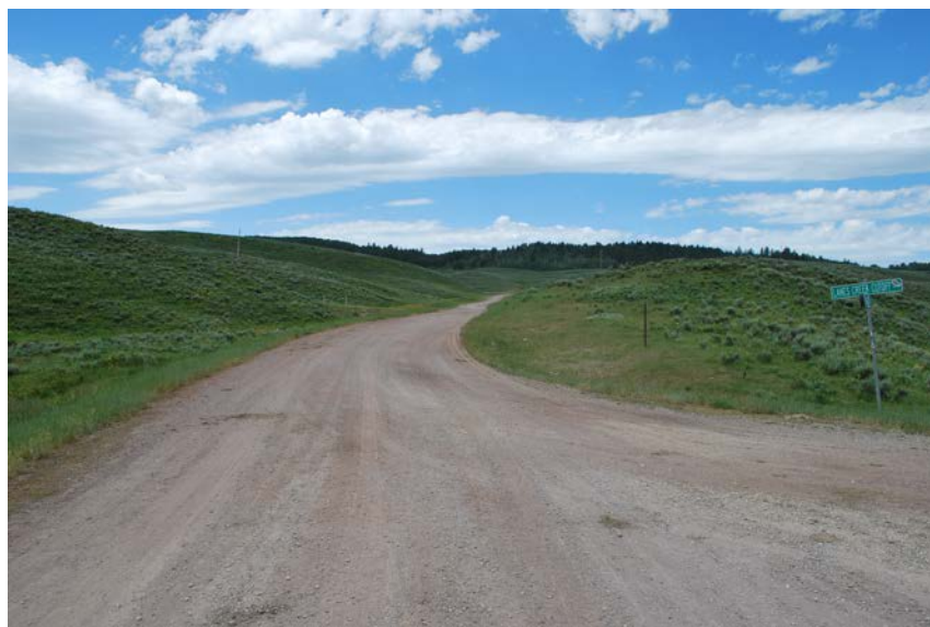
Figure 3-5. Photo 5—Lanes Creek Cutoff Road toward Lanes Creek Substation
