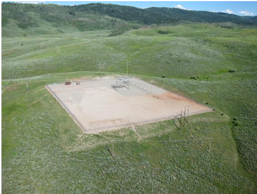
Figure 2-3. Existing Lanes Creek Substation
