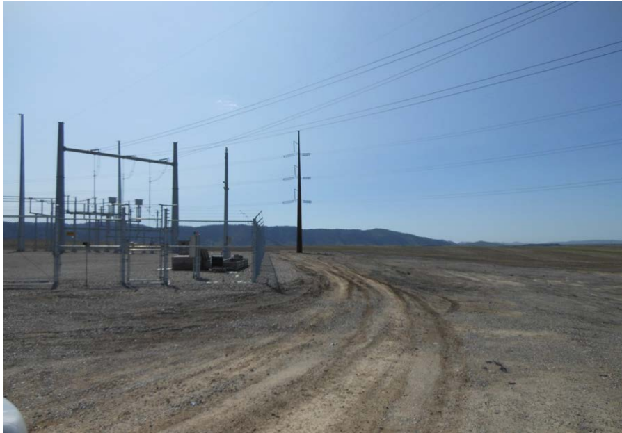
Figure 2-2. Area of the Proposed Hooper Springs Substation
