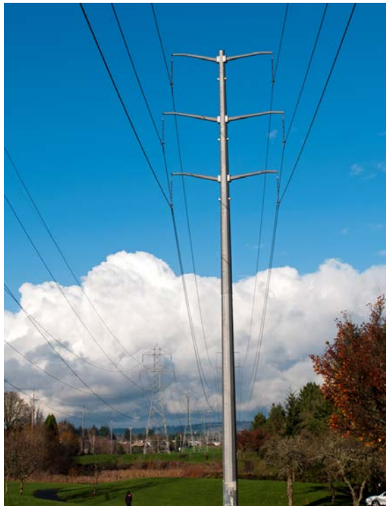
Figure 3-16. Typical Double-Circuit Transmission Line
