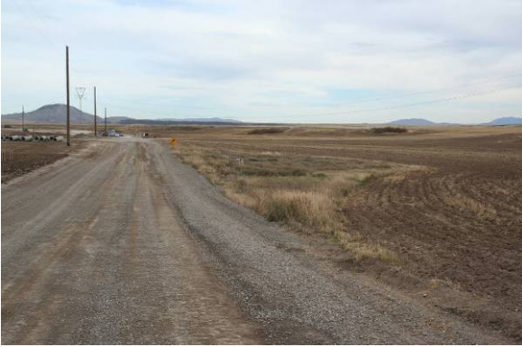
Figure 18 View north along 3-Mile Knoll Road near location where the substation would be built (to left of photograph) and transmission line would head east.
