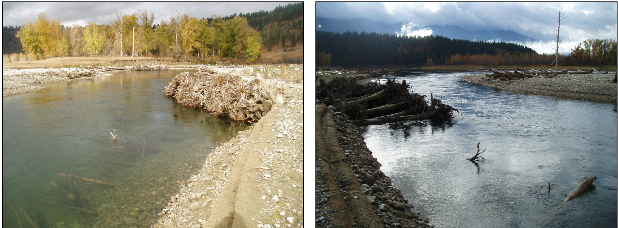
Figure 2-7. Type 1 wood structure immediately after construction.
