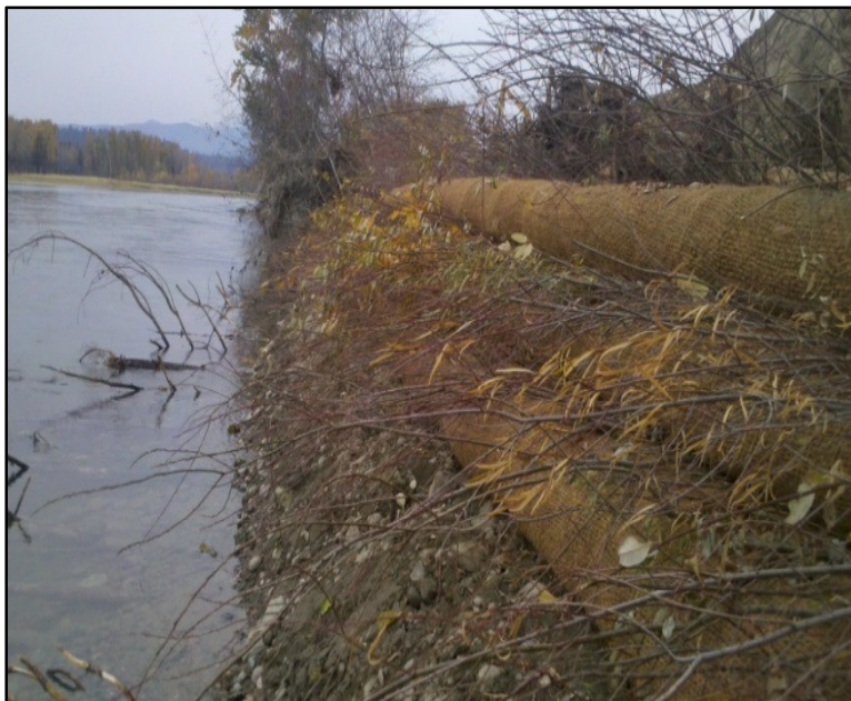
Recently completed soil lifts
