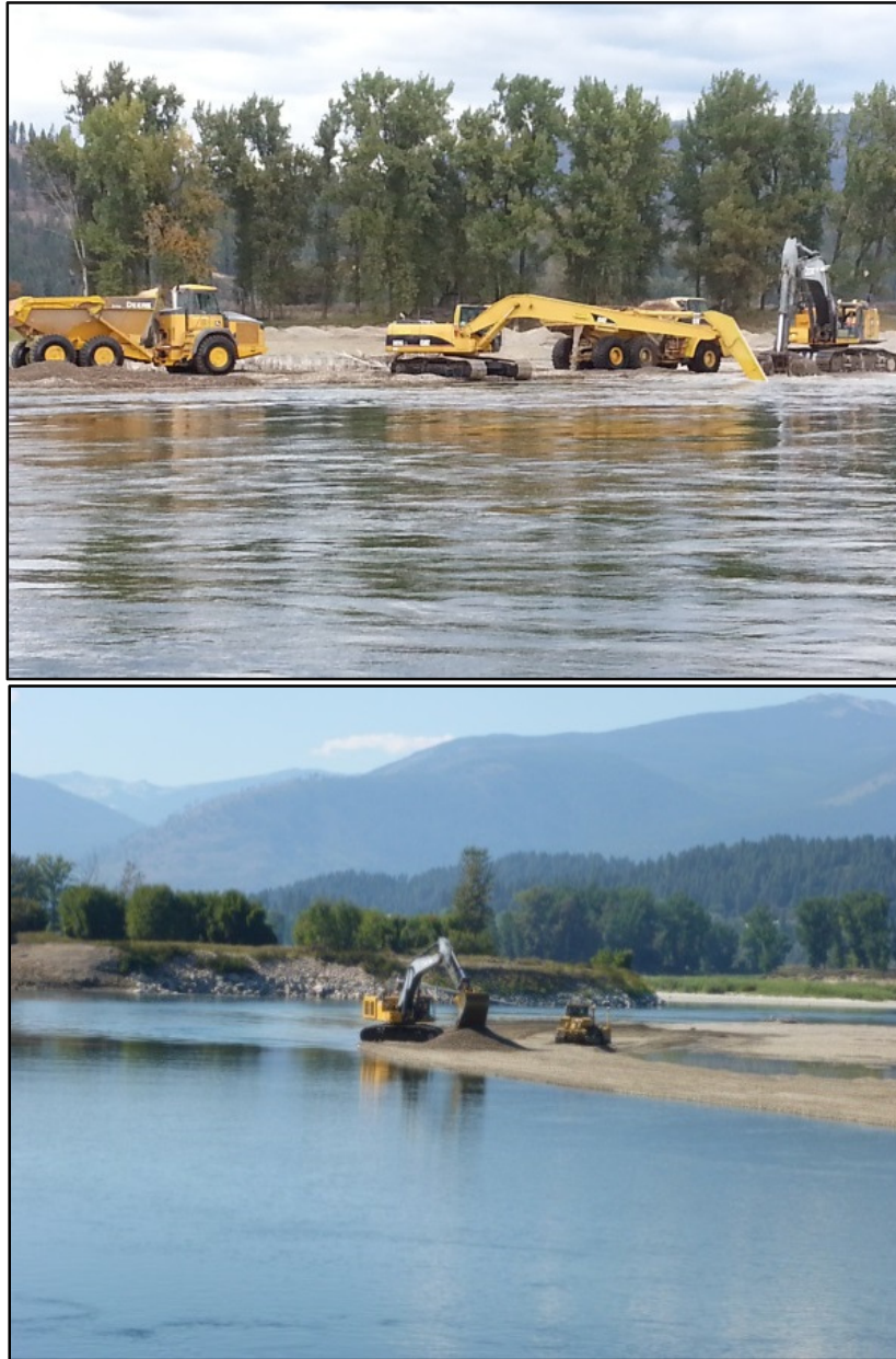
Figure 2-4. Examples of Pool Excavation
