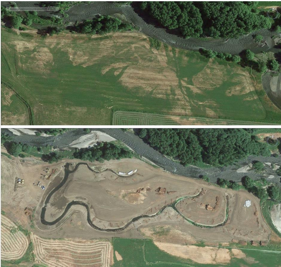
Figure 10 Short-term impacts to a floodplain during restoration project showing conditions before (upper photo) and during (lower photo).
