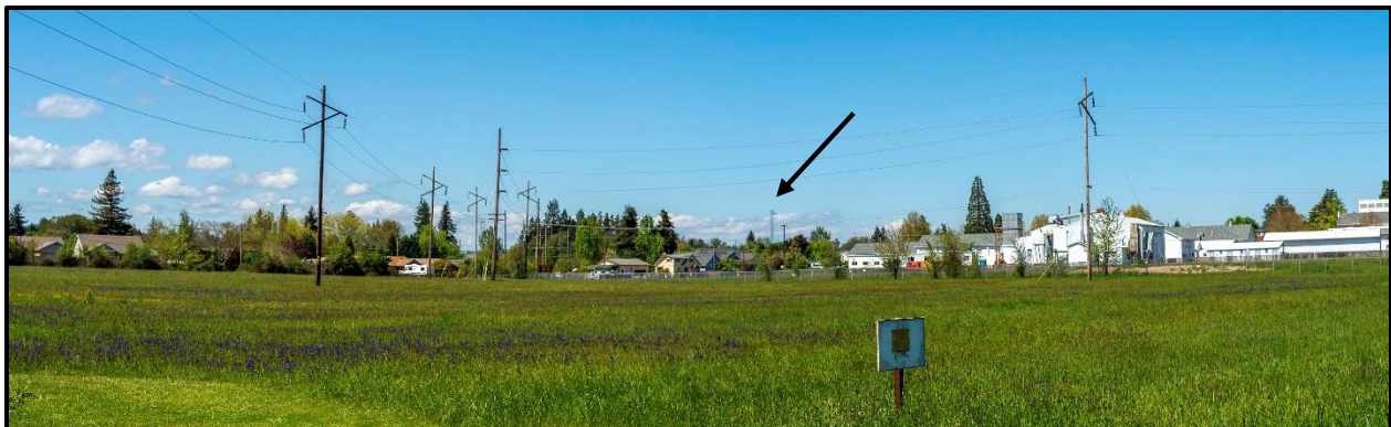
Photograph 3-31. View of the communications structure within the BPA Albany Substation from Liberty Street (KVA 16), looking west.
