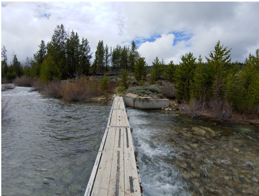
Figure 16 Area of Pettit Lake Creek streambed to be dewatered and impacted during weir construction
