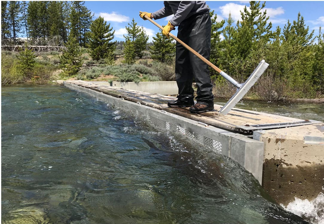
Figure 2 Pettit Lake Creek weir showing flat-plate slotted barrier for juvenile salmon capture
