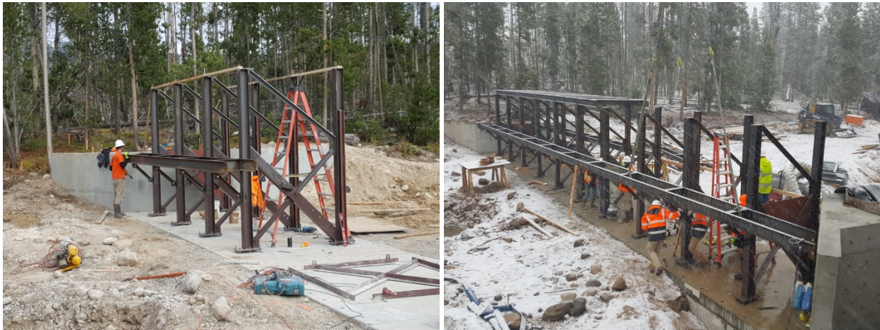
Figure 12 Example of similar bridge weir construction at nearby Redfish Lake Creek
