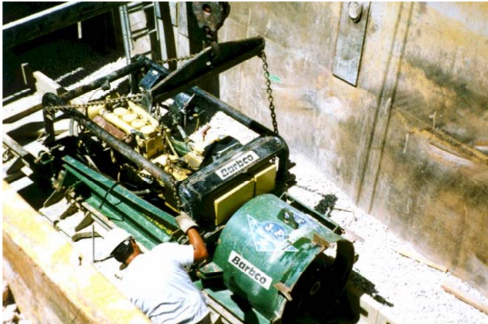
Figure 3-2: Typical Jack and Bore Set-up
