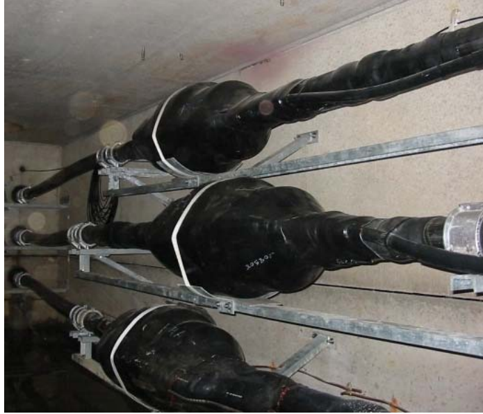
Figure B1-2 Typical Pre-molded 345kV XLPE Splice
