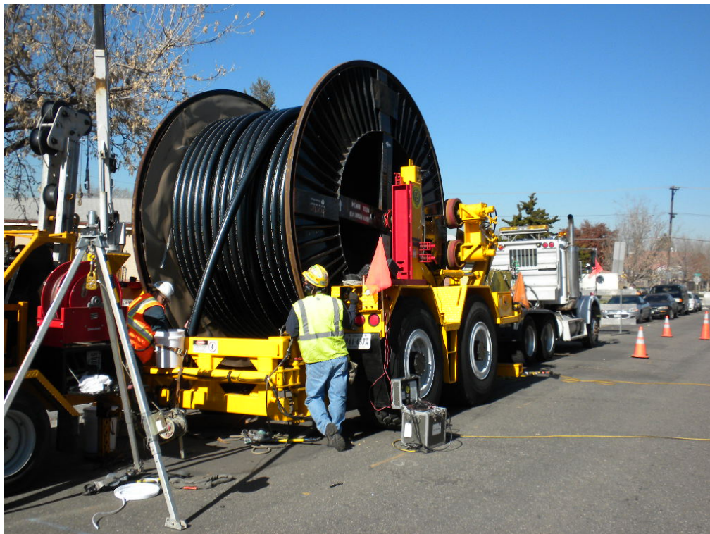
Figure 3-5: Typical Cable Pulling Set up
