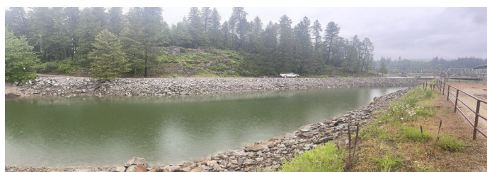
Albeni Cove Rip Rap showing the bank stabilization repairs FY 2022.
