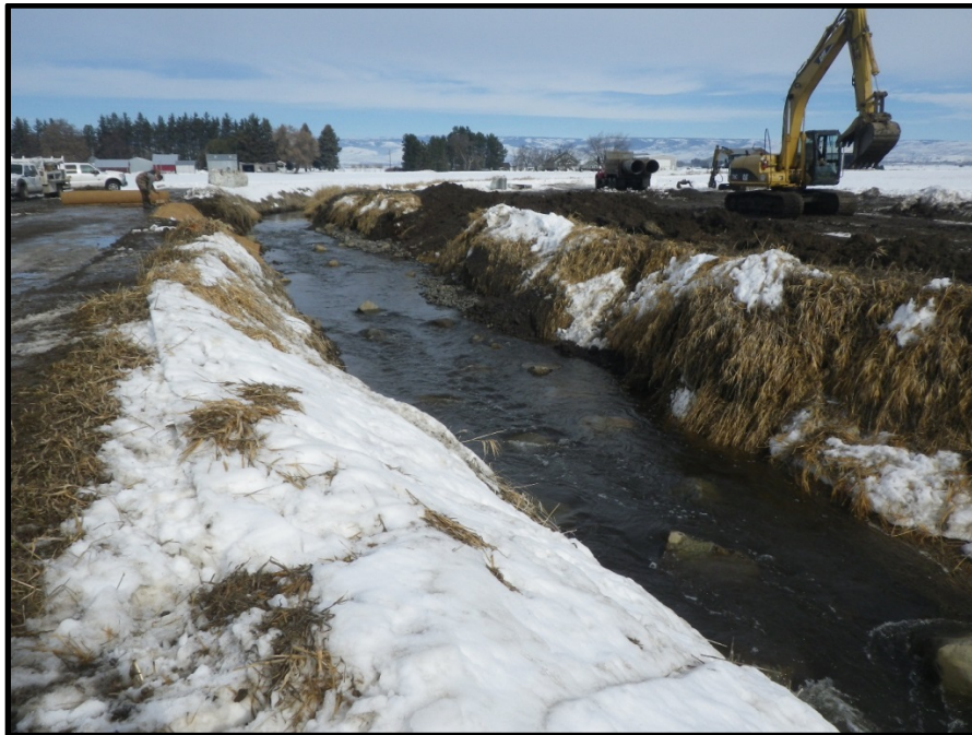
2017012(Caribou Creek)Diversion Removal After
