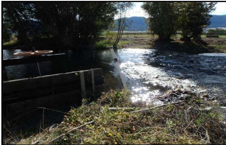
2017013: Tully Hill Barrier Removal and Grade Stabilization (After)
