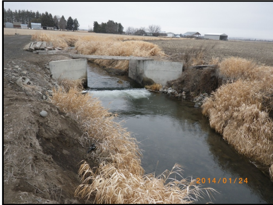
2017012(Caribou Creek)Diversion Removal Before
