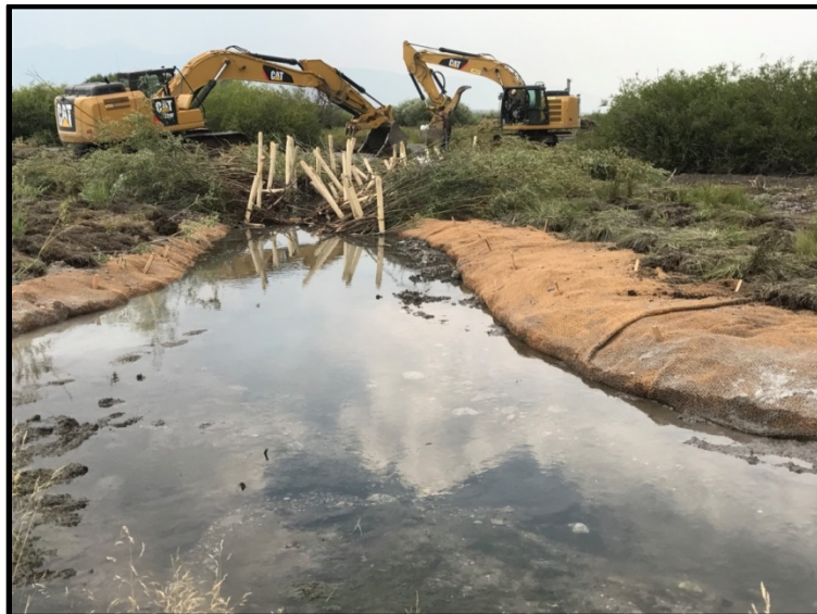
2017071(Lemhi_Fayle_Restoration)Bleeder Jam Installation
