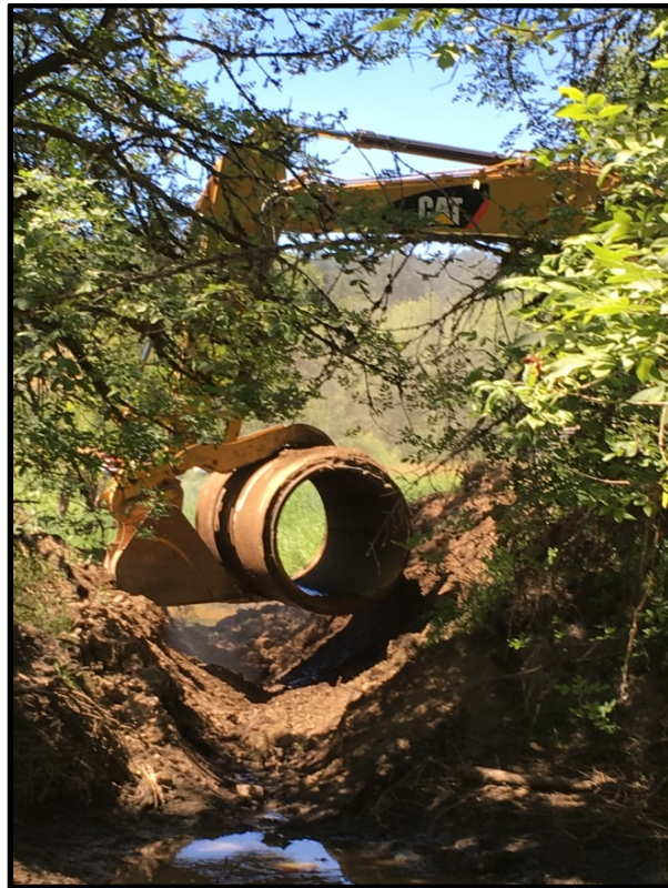
2017027(McCarthy Creek)Culvert Removal
