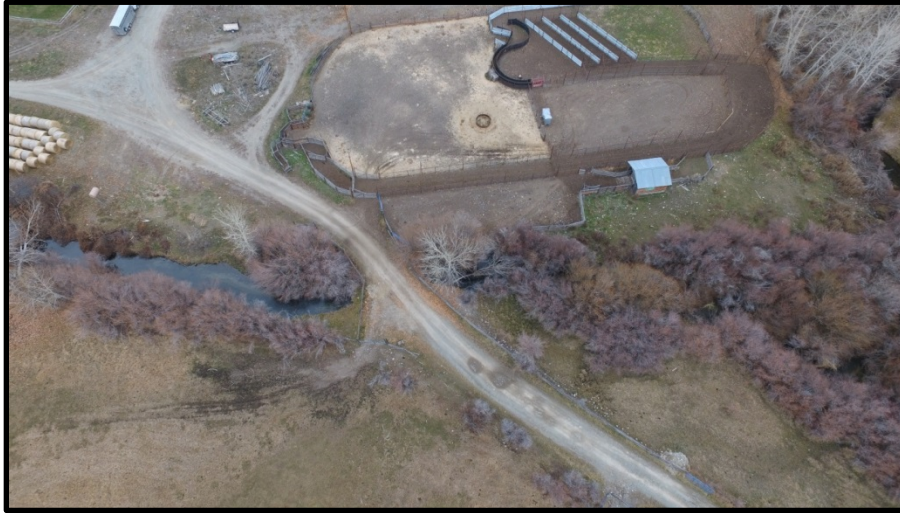
2017015 (Lemhi River Restoration) Bridge Replacement Before.
