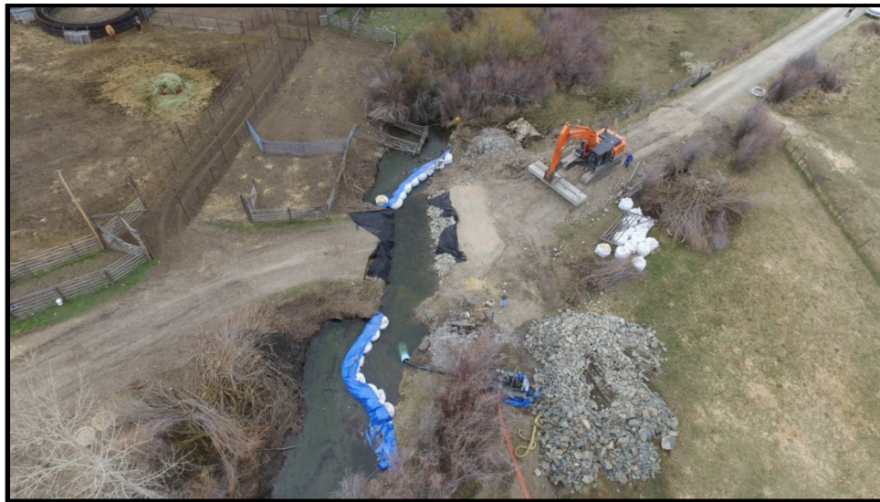
2017015 (Lemhi River Restoration) Bridge Replacement During.
