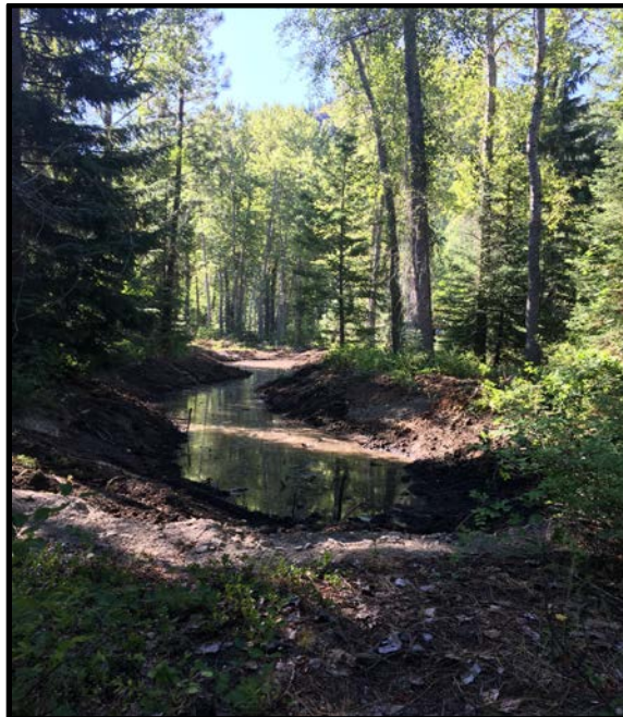
2017014: Newbry Meadows, Wetland replacement area excavated to subgrade before revegetation.
