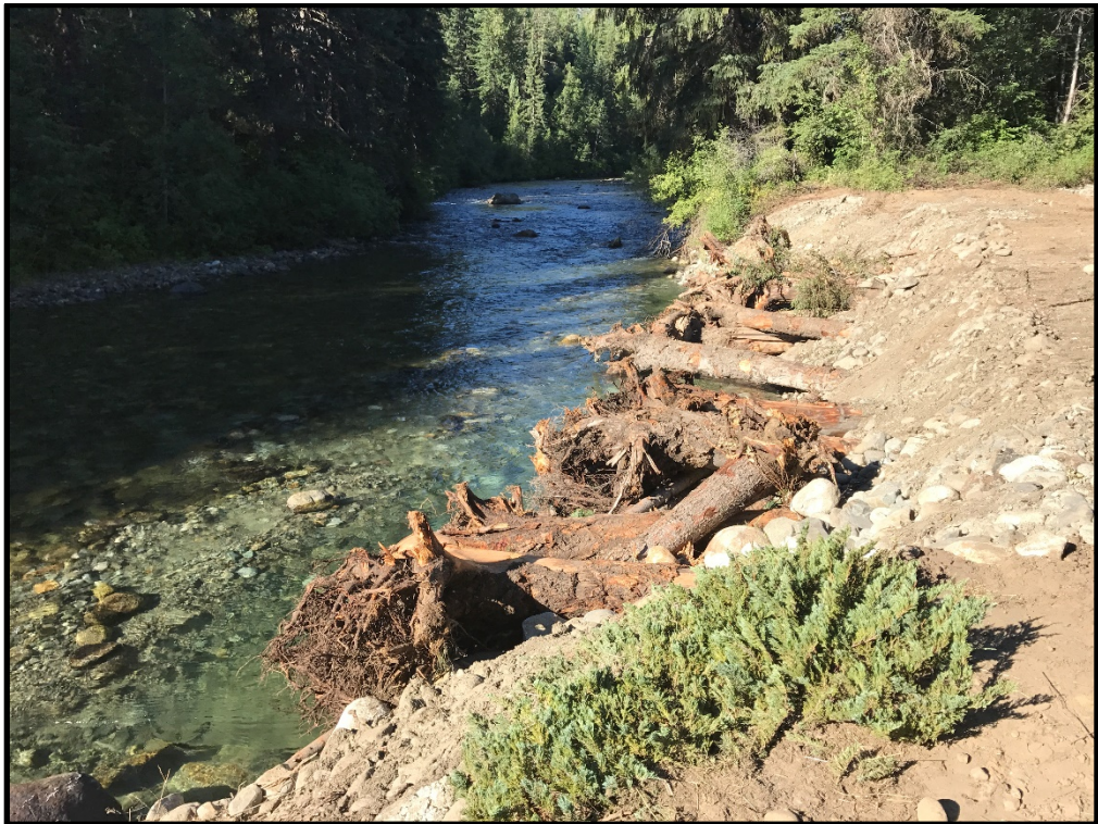
2017067(Horseshoe)Logjam Excavation After
