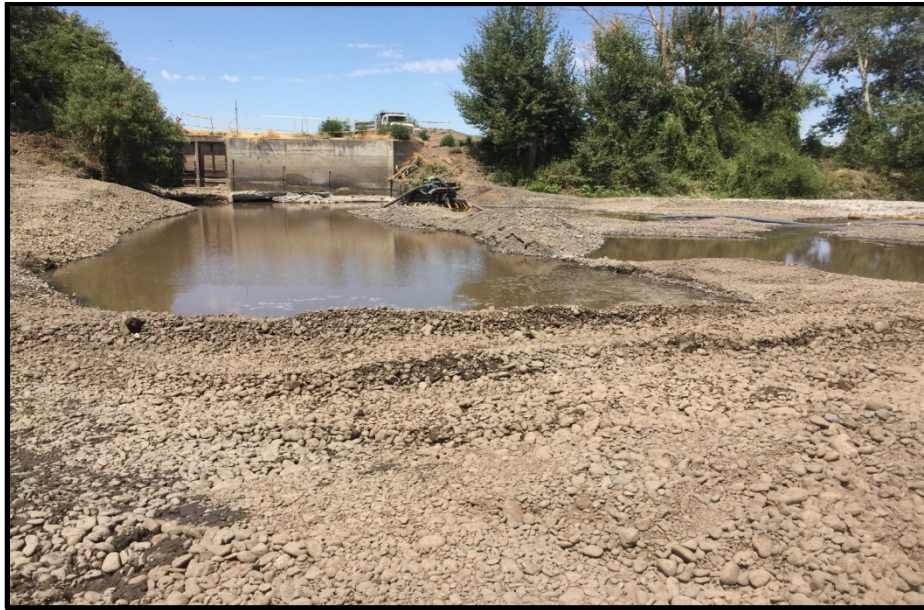
2017058- Dillon Dam Removal (After)
