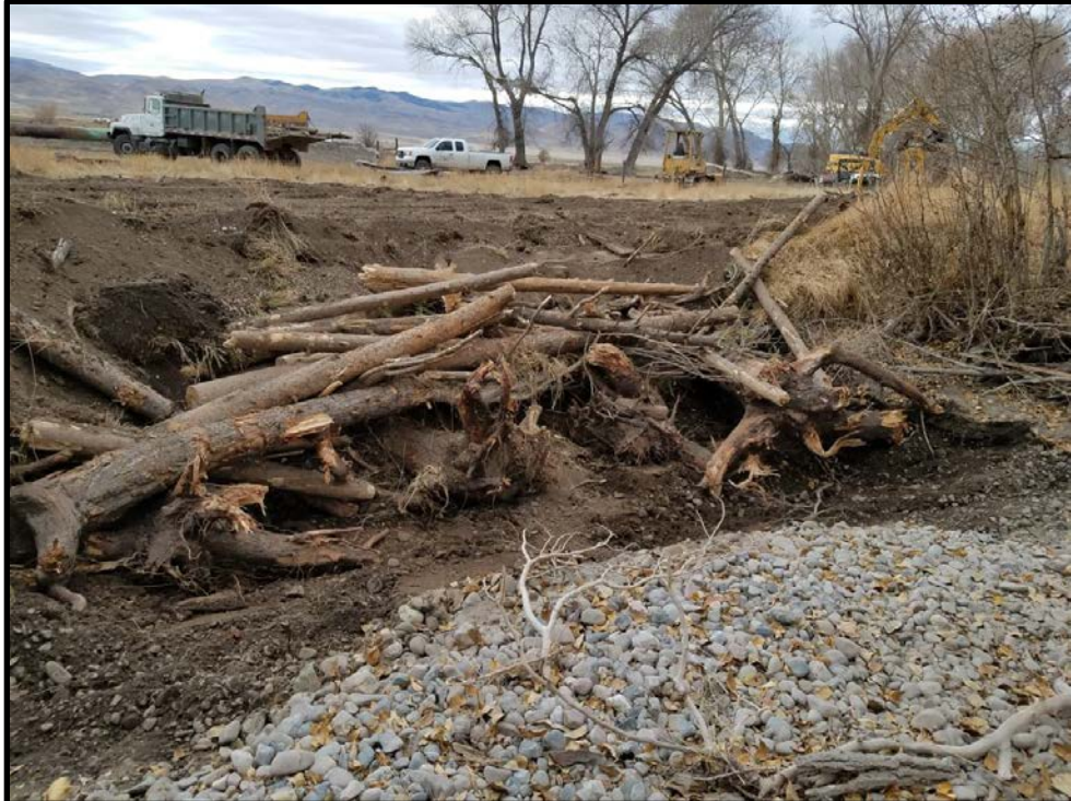
2017084 (Pahsimeroi Page) Installation of engineered log jam.
