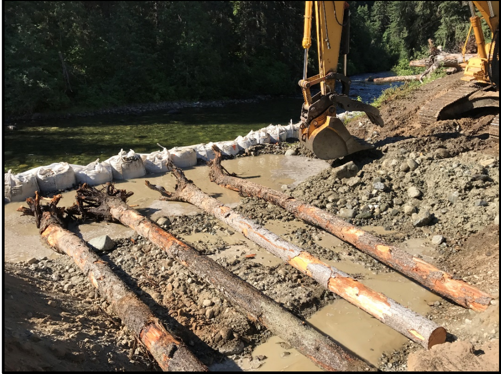
2017067(Horseshoe)Logjam Excavation During
