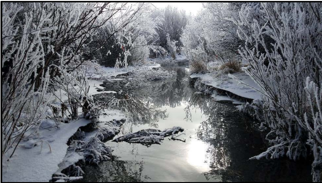
2017089 (Eighteenmile Creek Channel Reconstruction)
