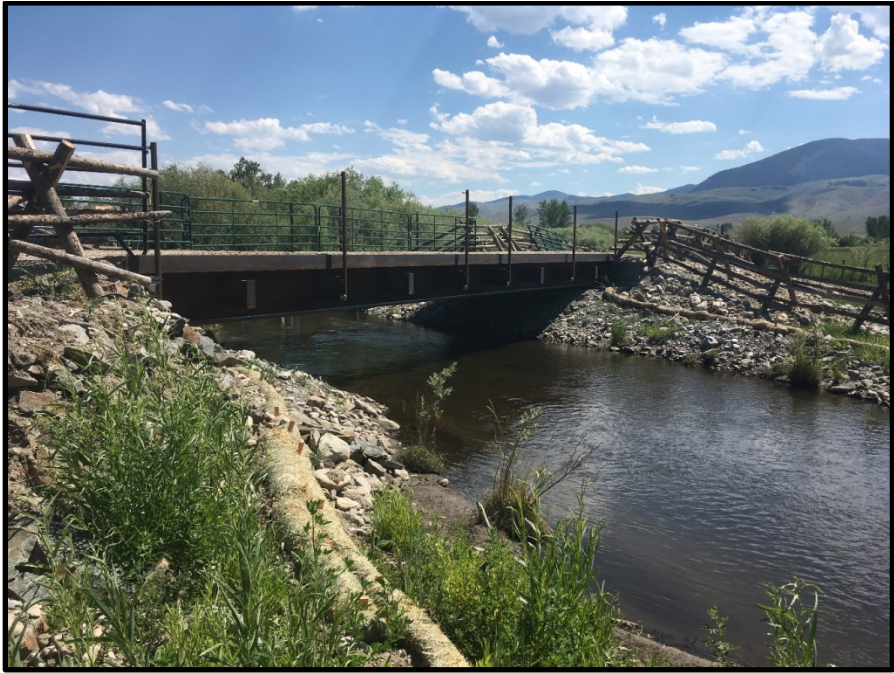
2017015 (Lemhi River Restoration) Bridge Replacement After.
