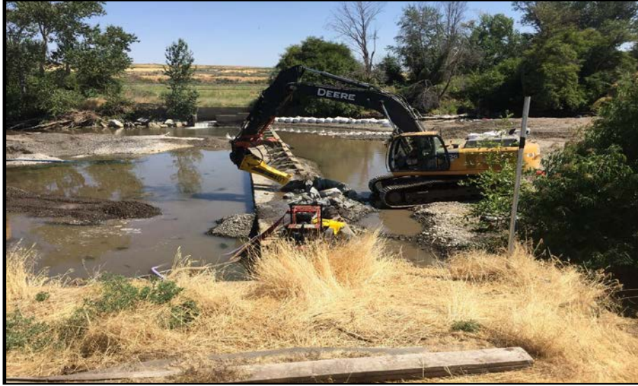
2017058- Dillon Dam Removal (During Construction)
