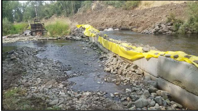
2017013: Placement of EcoBlocks caused 1 st turbidity Exceedance.
