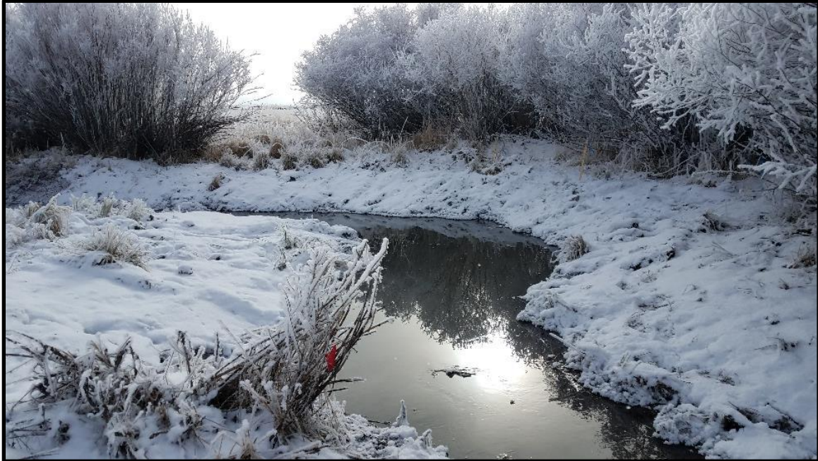
2017089 (Eighteenmile Creek Channel Reconstruction)
