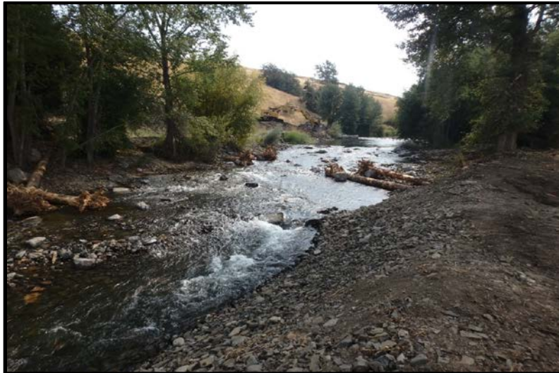
2017013: Tully Hill Grade Control Structures (After)
