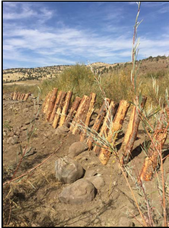
2016077(Dovenburg)Floodplain roughness features
