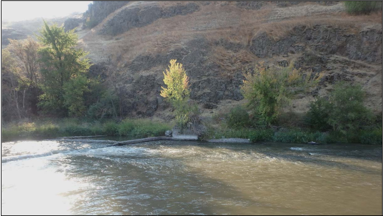
Photograph 1. Overview of the dam at 112° from the north side of the Umatilla River (18-106:27). 9/7/2018.
