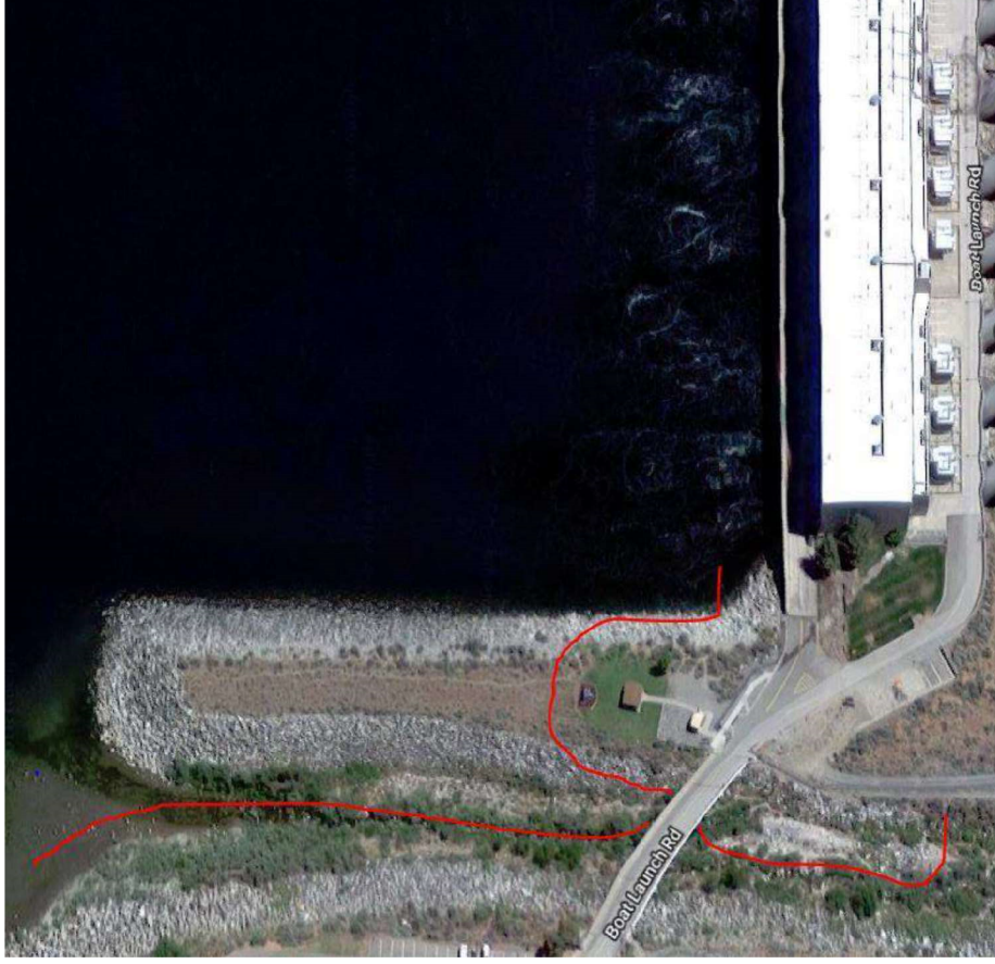
Figure 7-10. Aerial view of possible adult fish ladder at Foster Creek with secondary entrance in tailrace. Line in red shows site of adult fish ladder and entrances. Facility would be like that shown in Figure 7-9.
