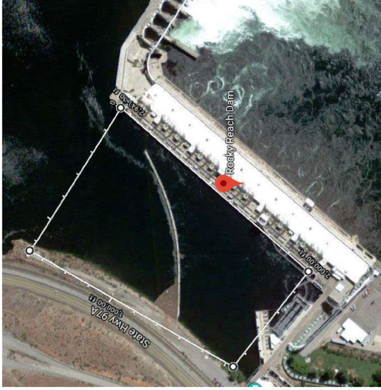
Figure 7-8. Aerial view of Rocky Reach corner collector. White line denotes effective forebay area (12 acres). Corner collector is in the lower left corner of the figure.
