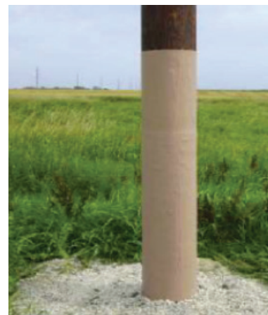
Figure 9: Heavy-duty coating applied to wood pole
