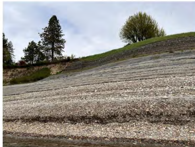
Figure 4. 45-FE-1. Western end of slope protection.
