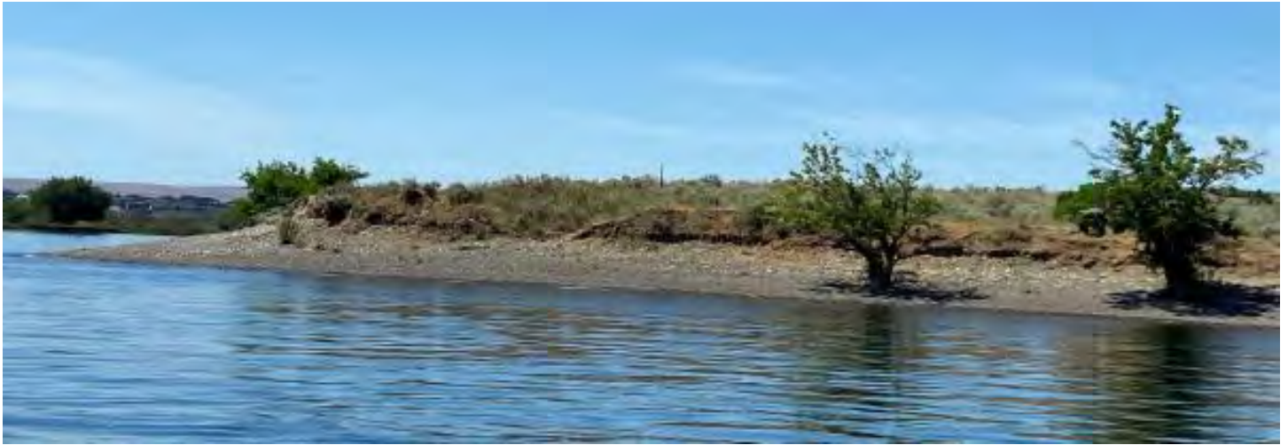
Bank erosion above cobble beach
