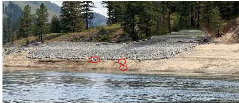
Figure 1. 45-ST-437 stabilization site. Note the large rocks circled in red that migrated downslope.
