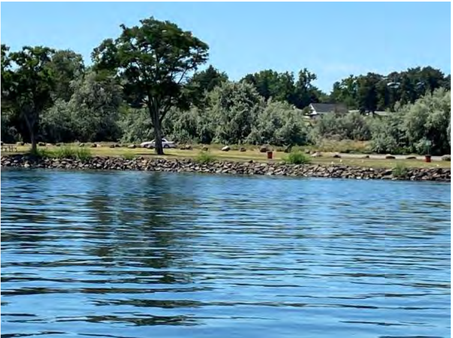
Bank stabilization riprap and willow plantings
