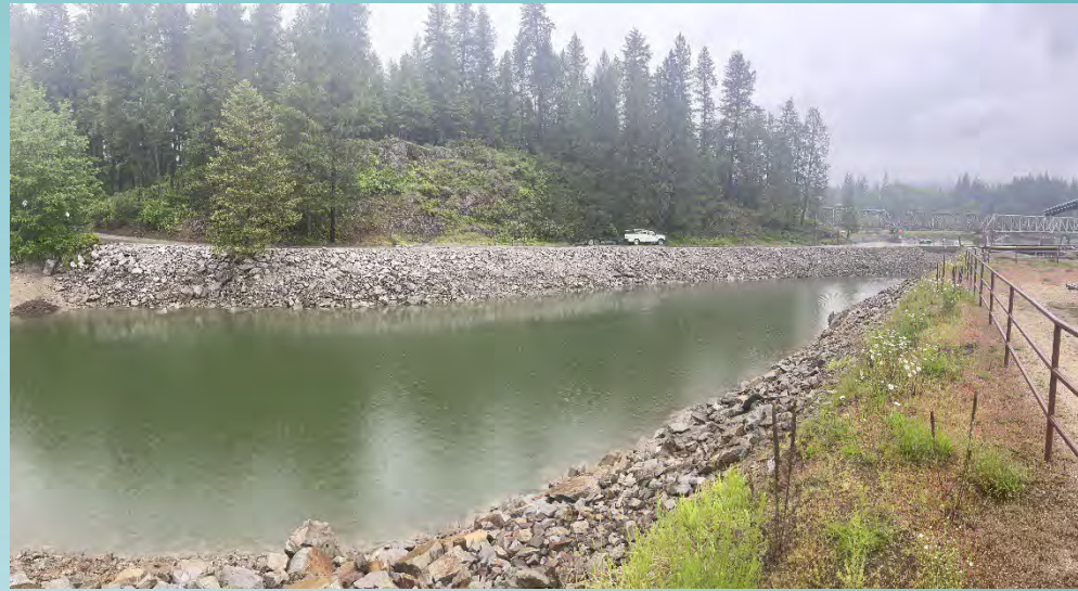
Rip Rap After
