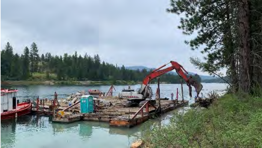
Figure H-4. Contractor's barge and equipment placing material.
