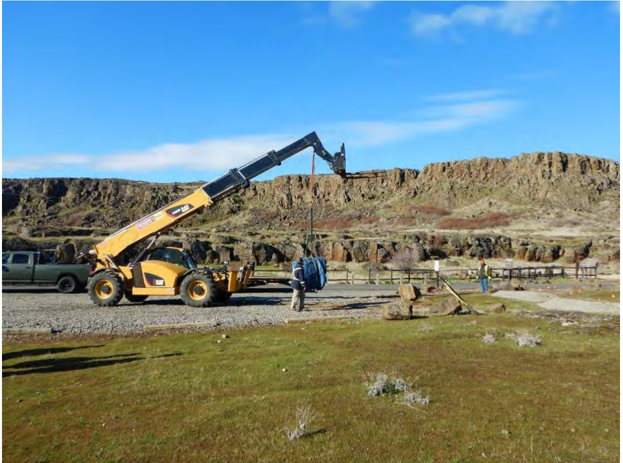
Figure E-2. Contractors place two petroglyph boulders along the Temani Pesh-wa trail in Columbia Hills Historical State Park, Washington, close to where the boulders were originally located before they were moved to Fort Vancouver in 1957.
