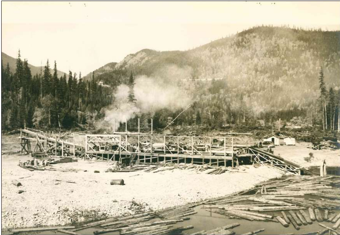
Figure 5 Sawmill on Egg Island in the Hungry Horse Reservoir flowage area. Source: BOR Project History, 1947, National Archives, Denver.
