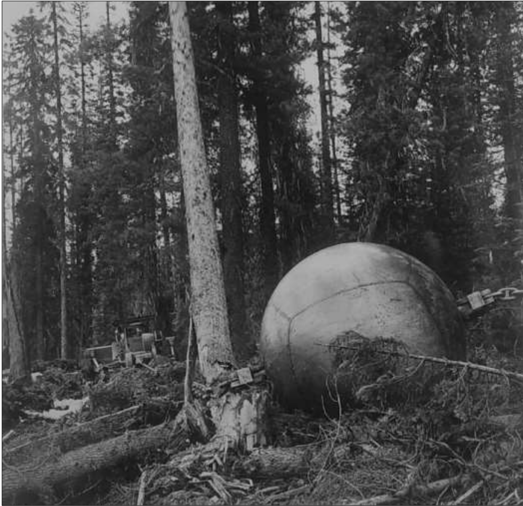
Figure 17 Highball clearing timber. Source: BOR Project History, 1950, National Archives, Denver.
