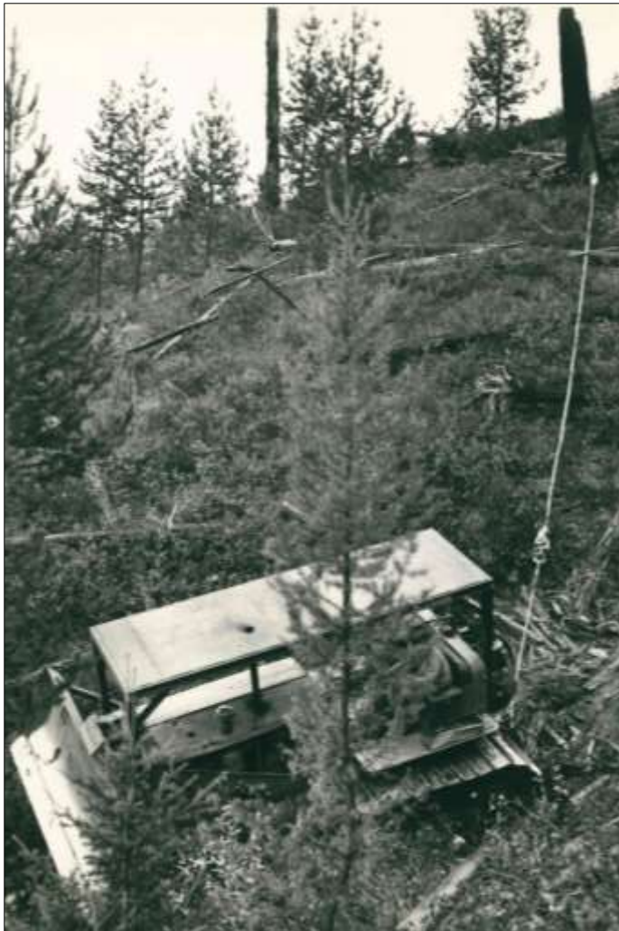
Figure 14 Cable attached to tractors to remove snags. Source: BOR Project History, 1948, National Archives, Denver.
