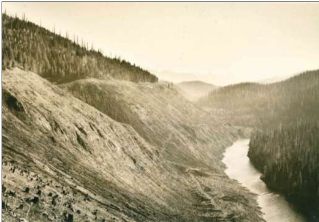
Figure 6 Canyon clearing. Source: BOR Project History, 1947, National Archives, Denver.
