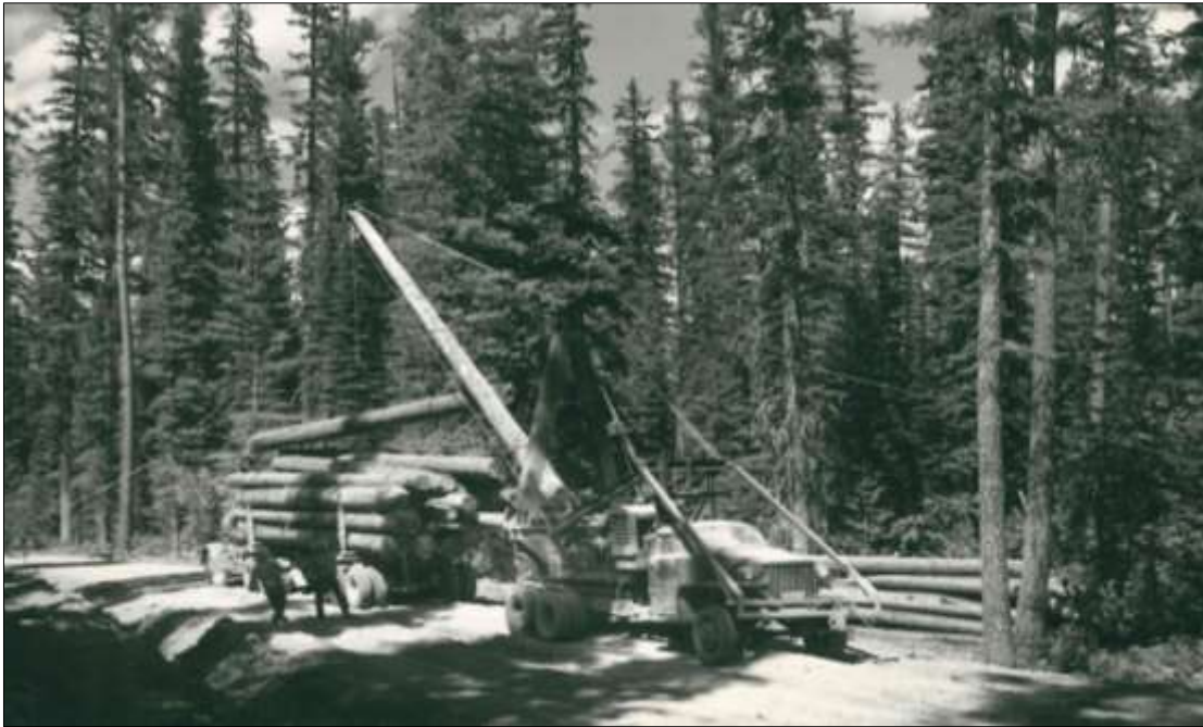
Figure 24 Loading a logging truck. Source: BOR Project History, 1952, National Archives, Denver.
