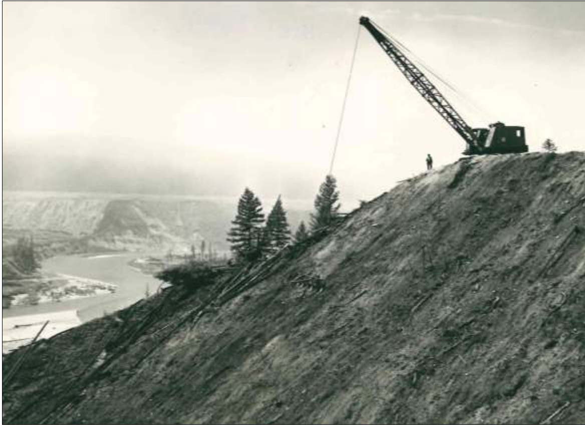
Figure 20 Wixon & Crowe clearing with a specially designed rake on steep terrain. Source: BOR Project History, 1951, National Archives, Denver.
