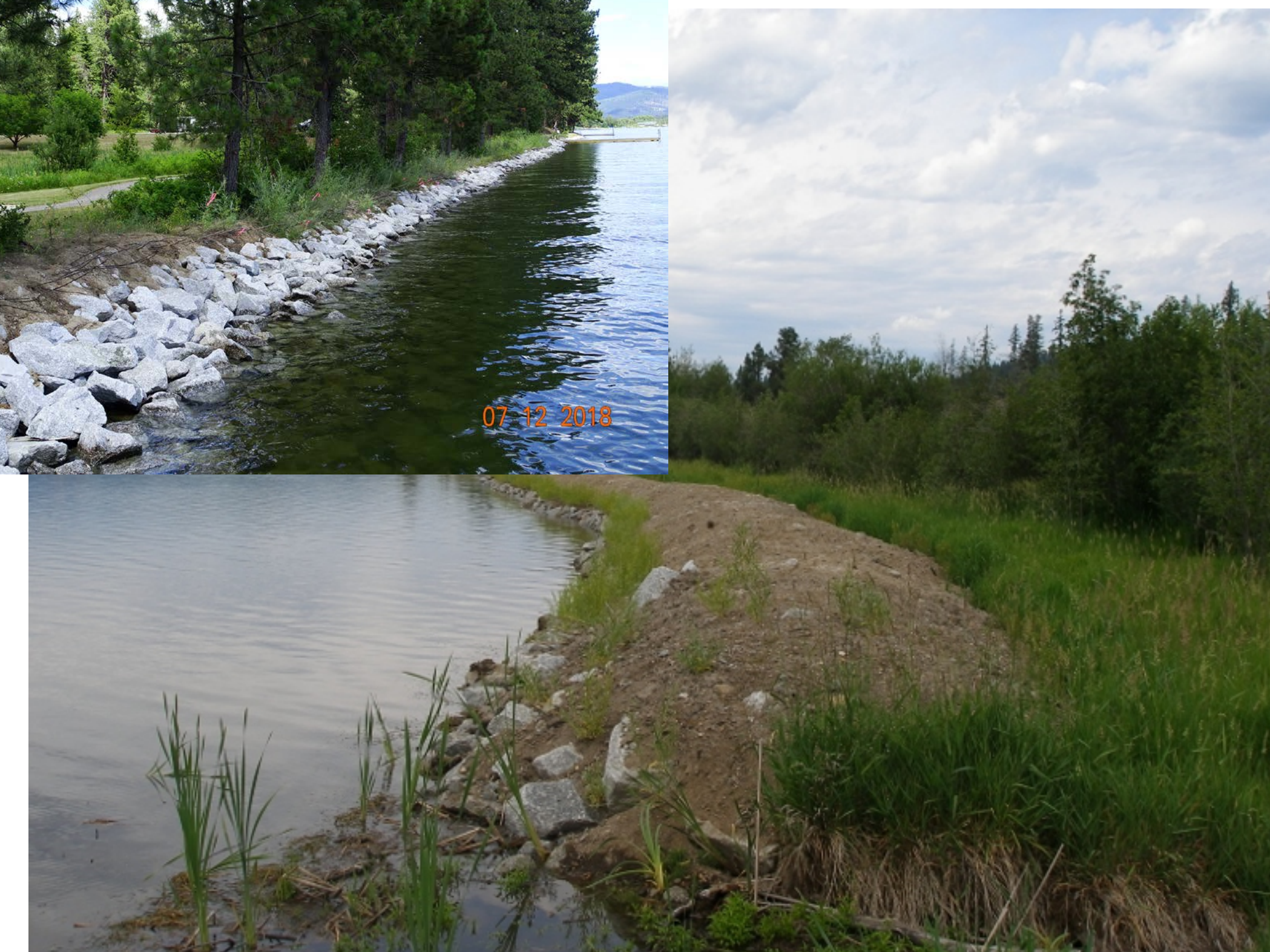
Priest River Stabilization
