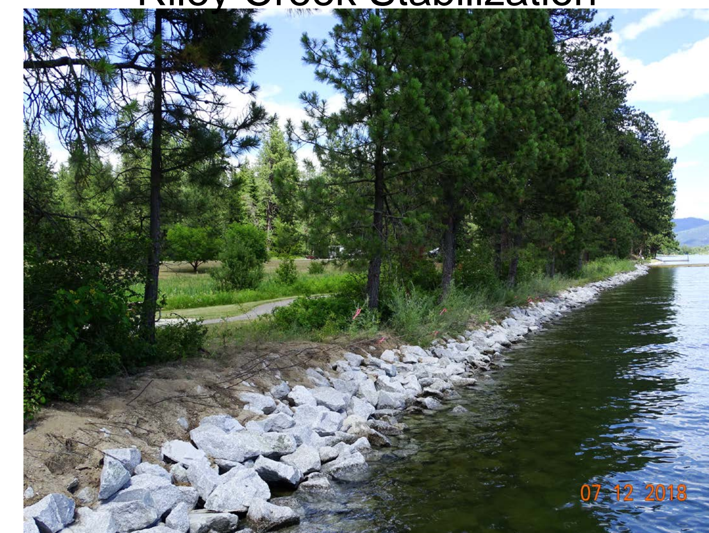
Riley Creek Stabilization
