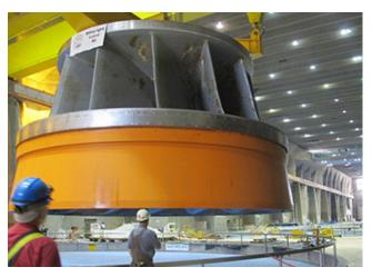
BPA and the Bureau of Reclamation are overhauling the Third Power Plant at Grand Coulee Dam in northeast Washington. Here, workers remove a 3,000-ton hydroelectric turbine that had been producing power since the 1980s. All six turbines in the third powerhouse will be refurbished in the next 10 to 15 years as part of a \$275 million project funded by BPA ratepayers.
