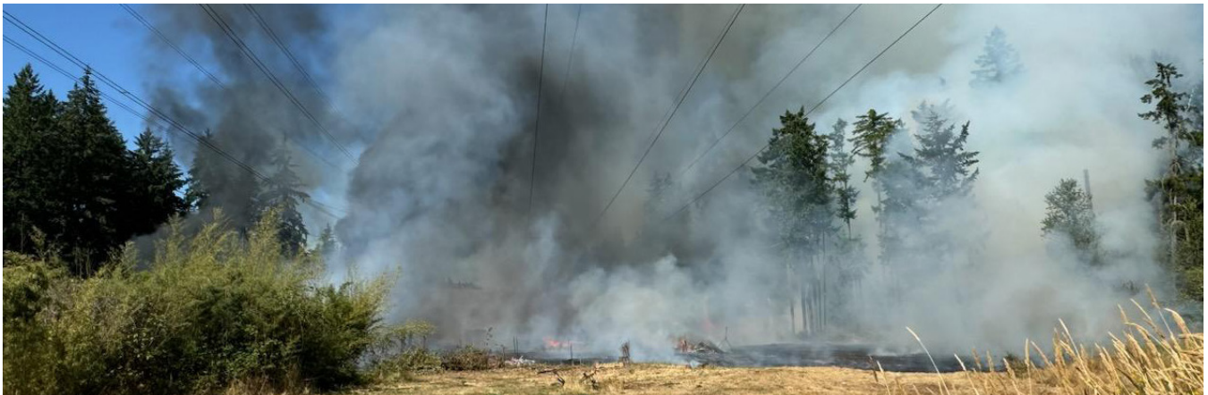
Smoke from a wildfire obscures the sun above a BPA substation.
